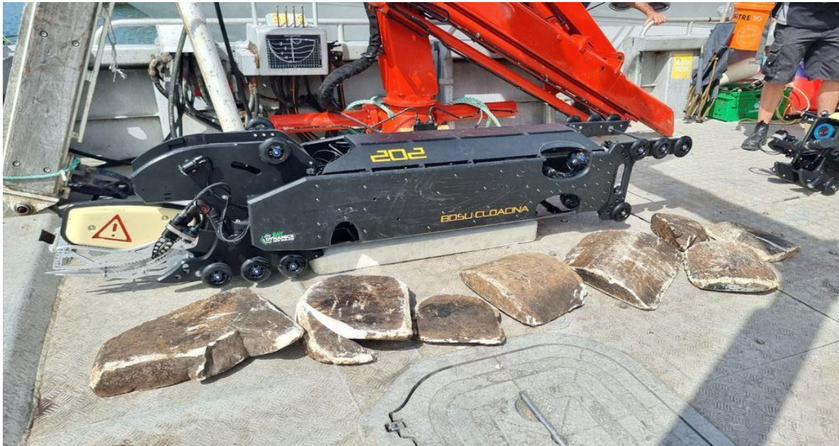
Photo 9: Grout Debris Removed on Day 2
