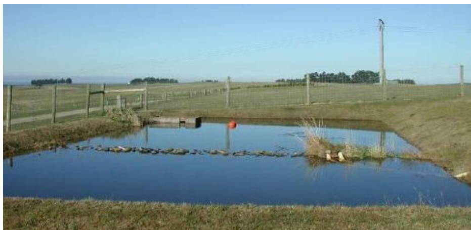
Photograph 5: Typical settling lagoon at Waikouaiti WTP
