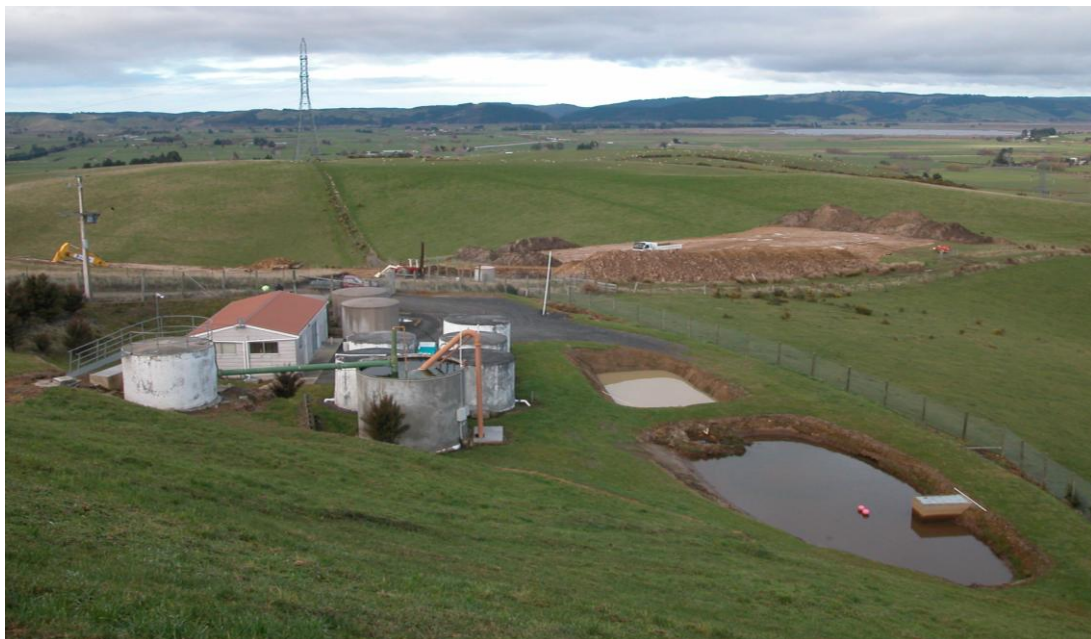
Photograph 1: Previous West Taieri WTP
