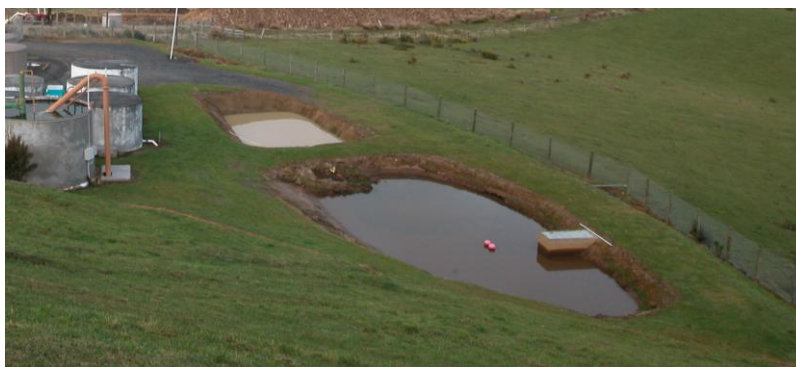
Photograph 4: Previous backwash/settling pond and drying pits at West Taieri WTP
