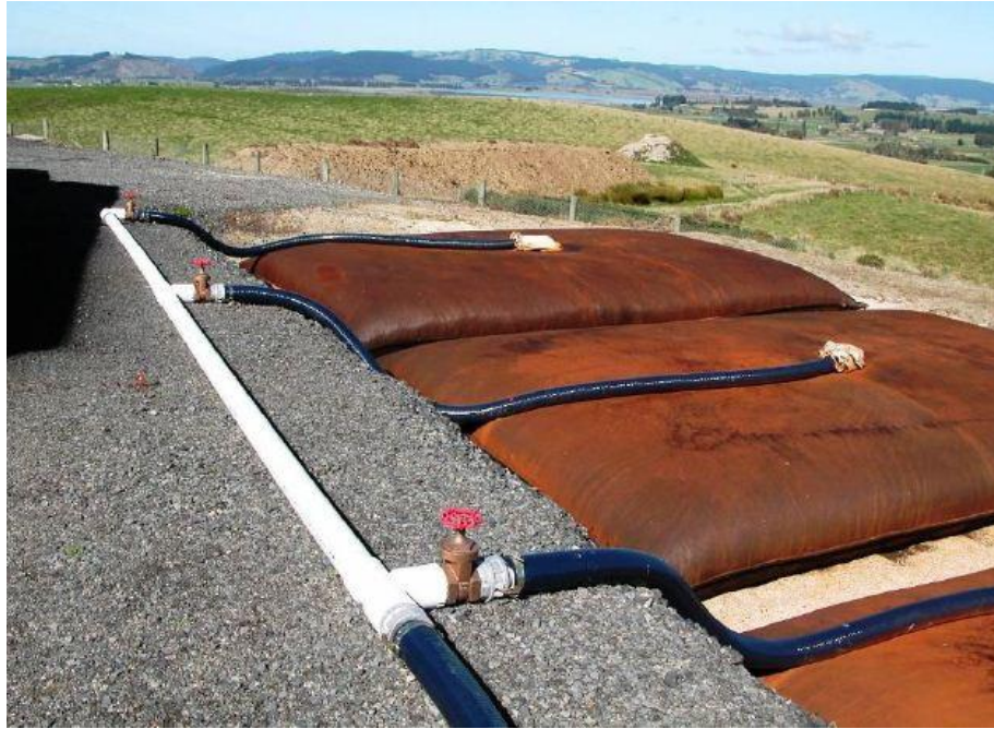
Photograph 6: Geobag System at West Taieri WTP
