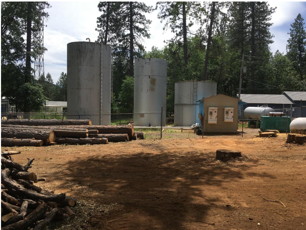
Photograph 2: "Two manually-operated storage tanks in poor repair (left) share a backyard with another partially-collapsed steel tank (right) next to this California system's treatment enclosure." Photo Credit: Susan Willis/ GHD
