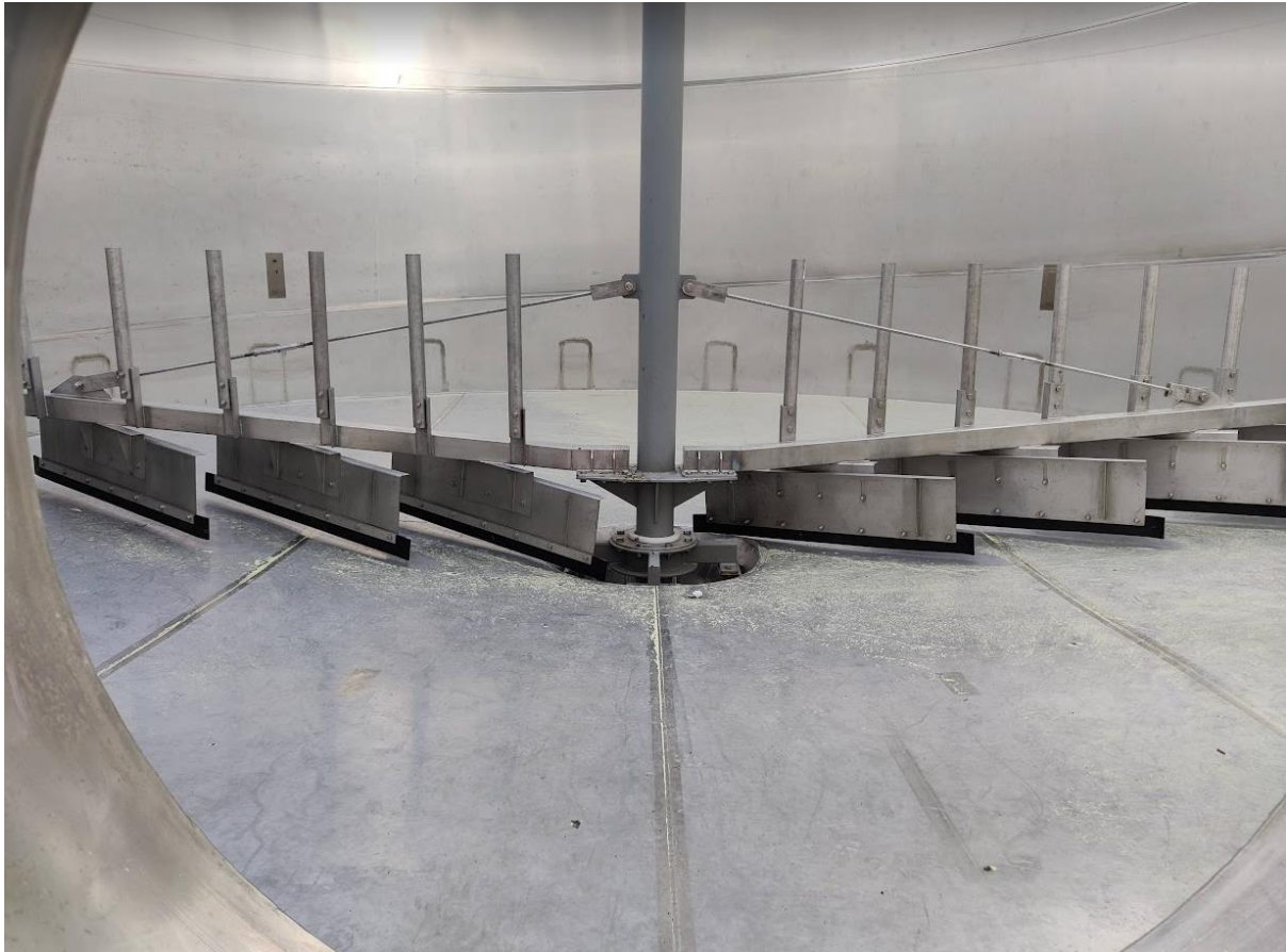
Photograph 1: An example of removing a confined space.
