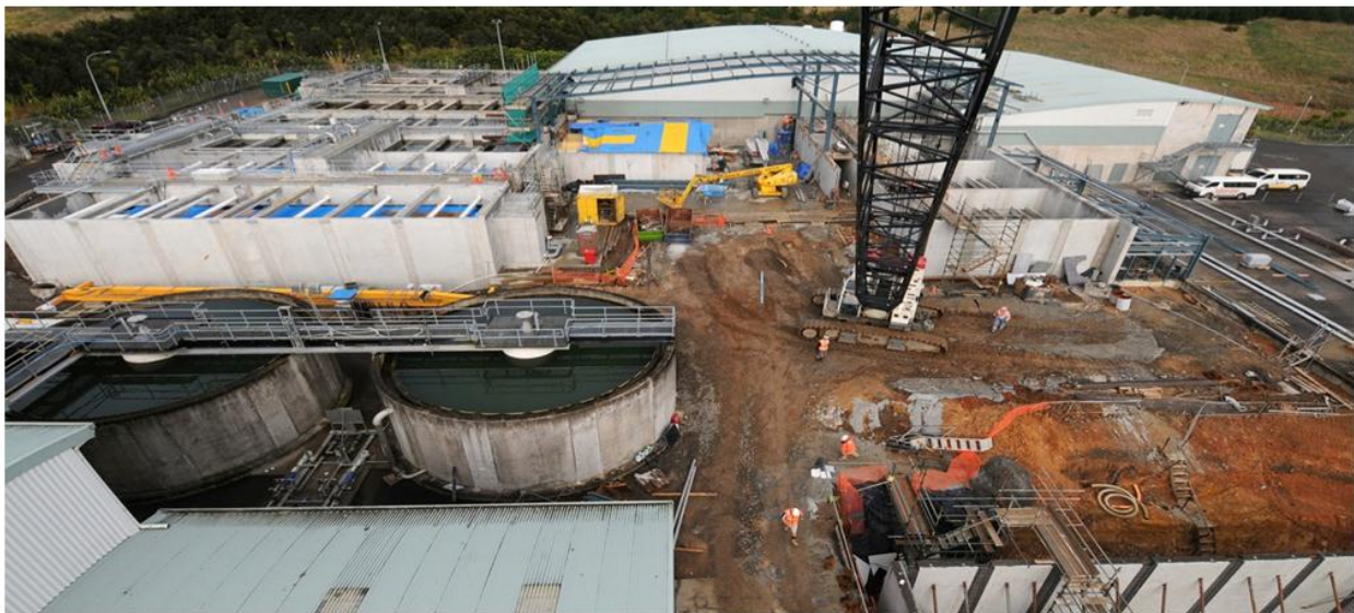
Photograph 2: The site during the construction phase
