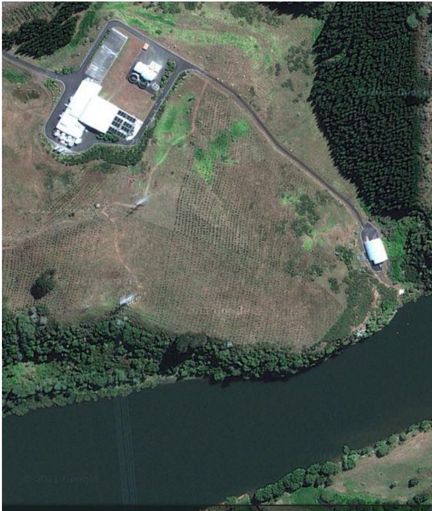
Photograph 1: Waikato Water Treatment Plant – Pre Expansion (75 MLD capacity)
