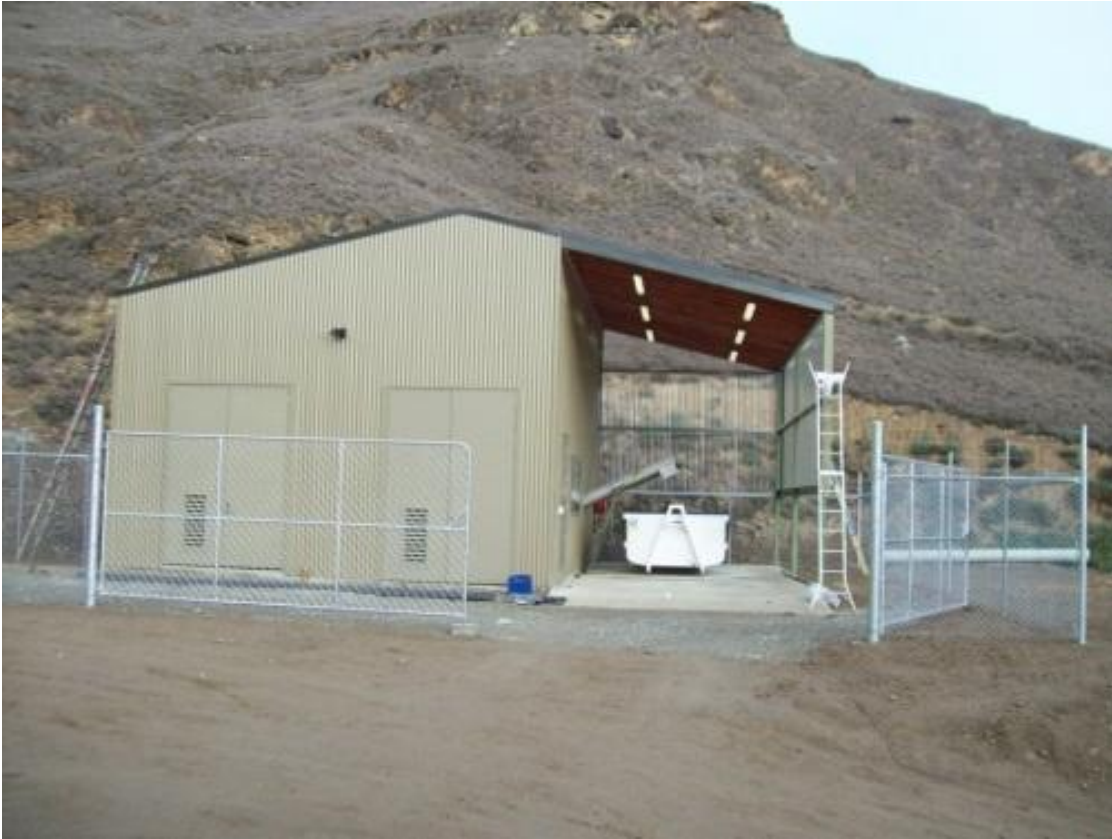
Photograph 3: Completed Sludge Dewatering Building
