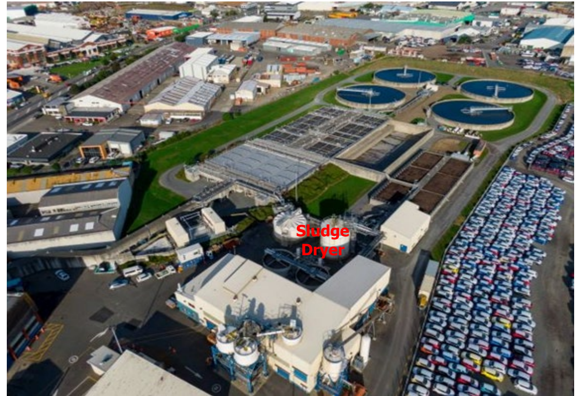
The natural gas fired sludge dryer at the Seaview Wastewater Treatment Plant, Lower Hutt City Council is up for replacement.
