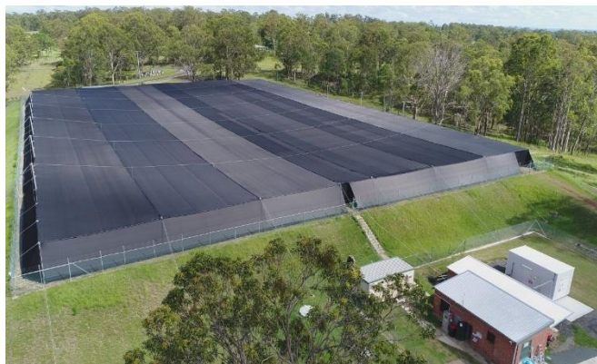
Rushforth Road Reservoir – exterior (Credit: Beca HunterH2O)
