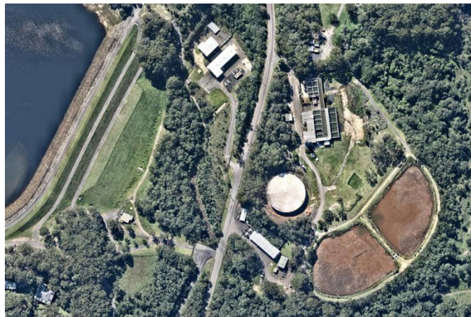
Mardi Water Treatment Plant (aerial) (Credit: Beca HunterH2O)
