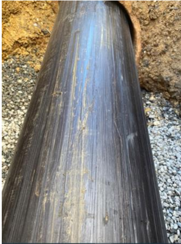
Figure 9: External condition of the new pipe post-slip lining (top of pipe).
