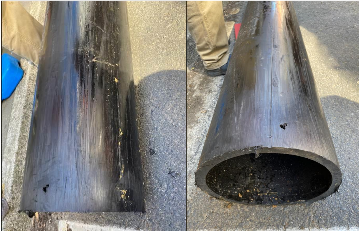
Figure 8: External condition of the three-meter long test section post-slip line.
