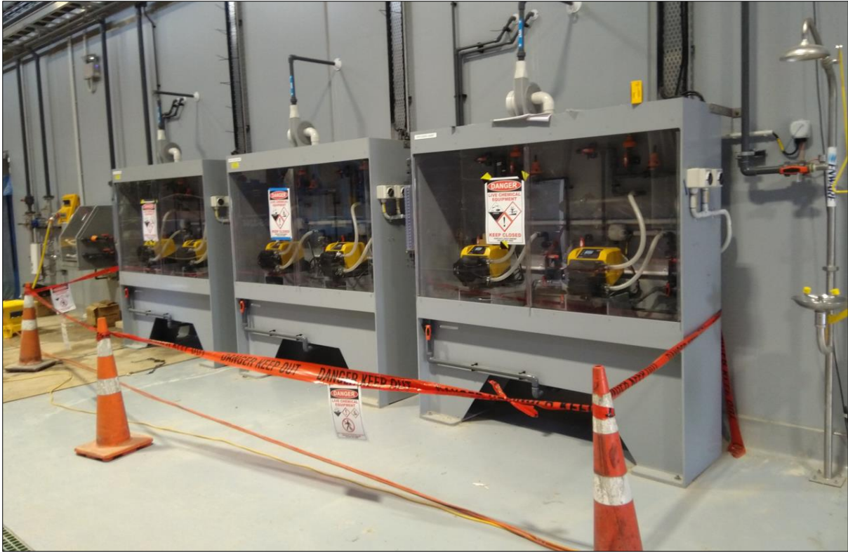
Figure 5 –Example of Commissioning Area Demarcation
