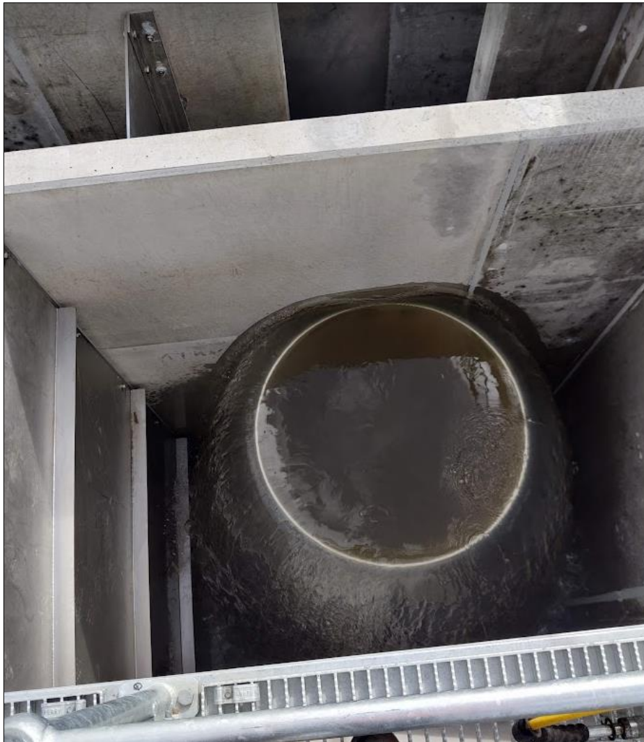
Figure 6 – The First Water To Enter The WTP
