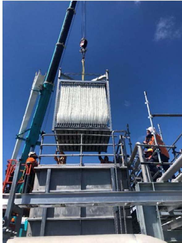
Figure 5: MABR Cassette Installation
