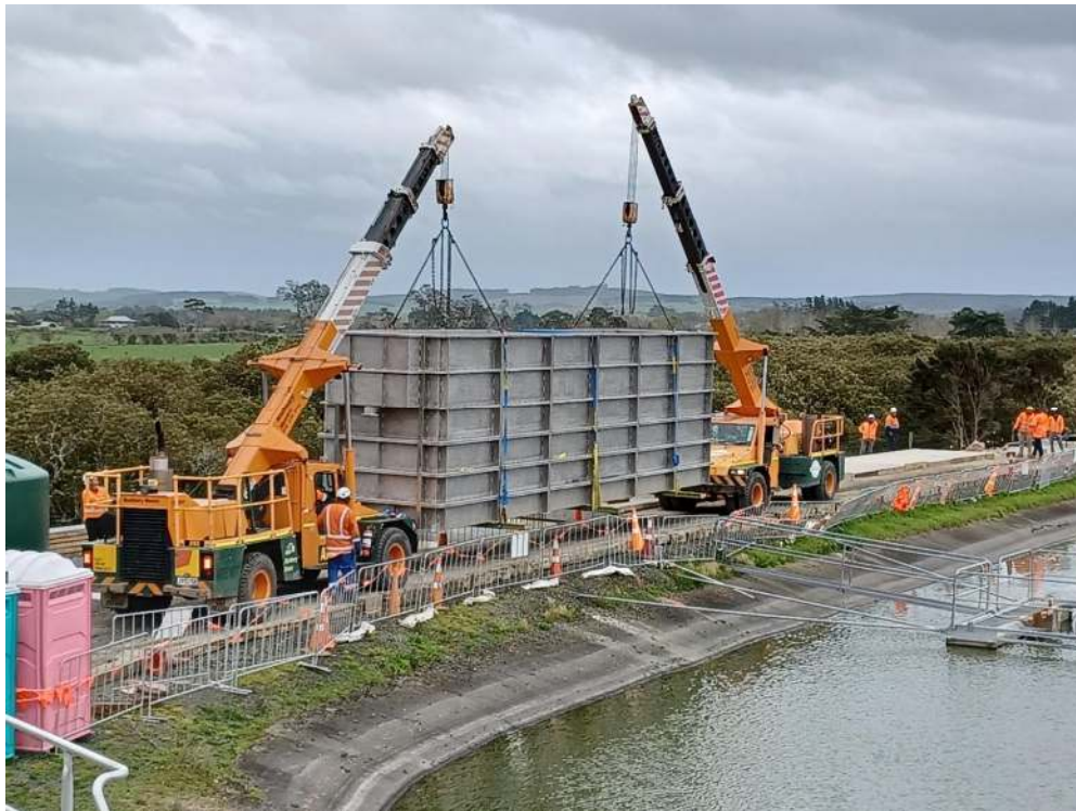
Figure 4: MABR Tank Installation
