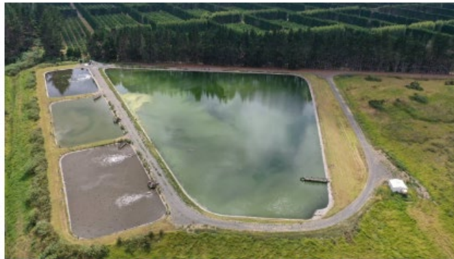
The Taipa wastewater treatment plant serves Taipa (pictured), Mangōnui, Coopers Beach and Cable Bay. Photo / Petrina Hodgson
