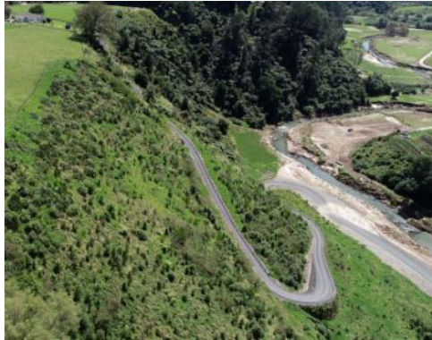
Photograph 3: Waiāri access track.
