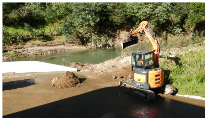
Photograph 13: Clean-up operation in progress.
