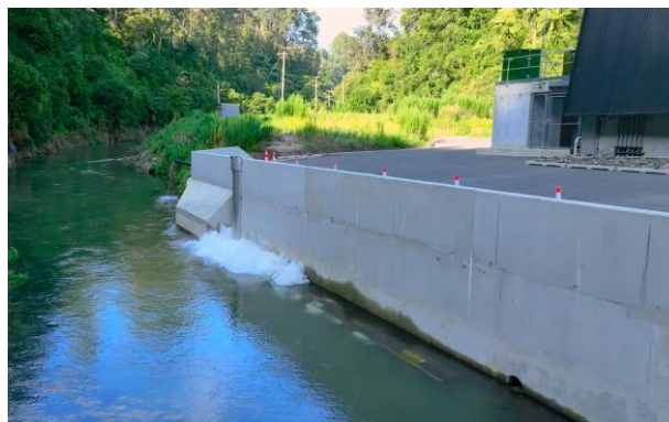
Photograph: Lower access platform.
