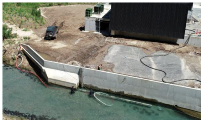
Photograph 11: Divers installing spool pieces to the TCC screens.
