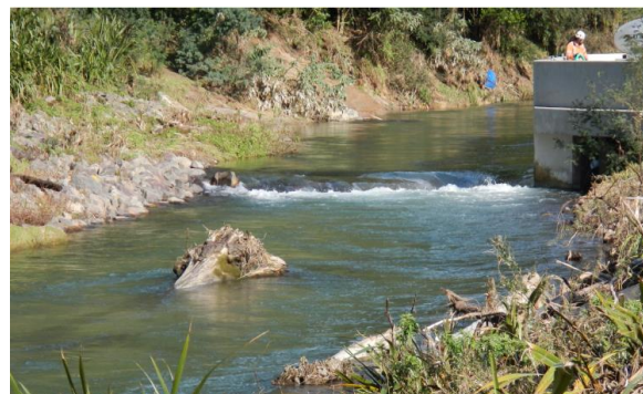
Photograph 9: Typical debris residue following the flood events.
