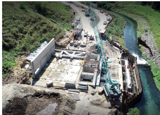
Photograph 5: Ground improvements and deflector wall under construction.
