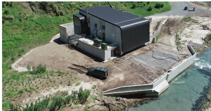
Photograph 12: Partly cleared silt from lower platform.
