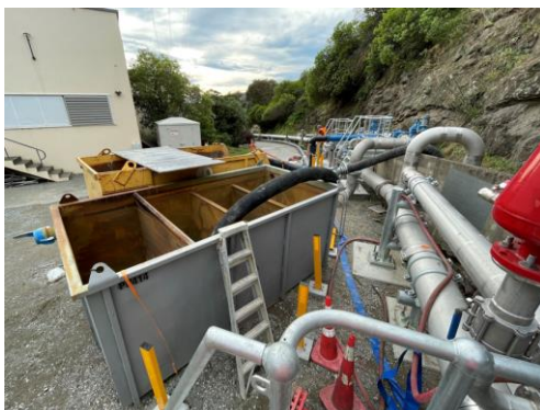
Figure 5: Overflow capture system
