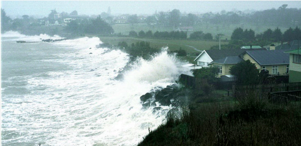
Rough seas at Timaru. Credit: NZ Herald ( https://niwa.co.nz/natural-hazards/hazards/coastal-storm-inundation )
