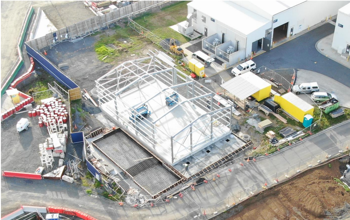
Figure 8: Construction progress of building and tank slab formwork
