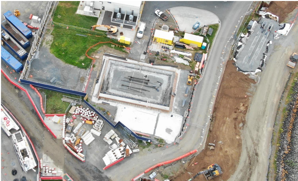
Figure 7: Drone photo overview of RWP building slab and tank slabs.
