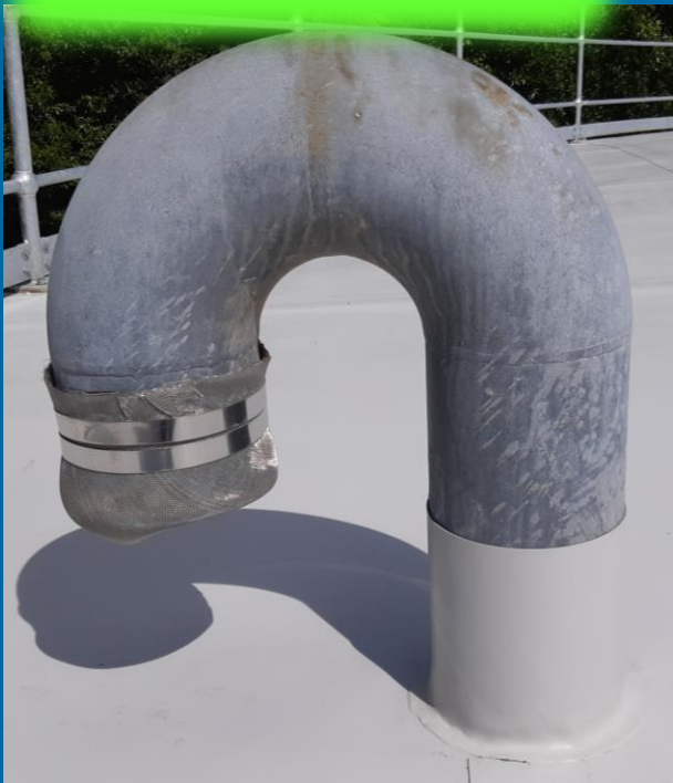
Air Vent Mesh installation
