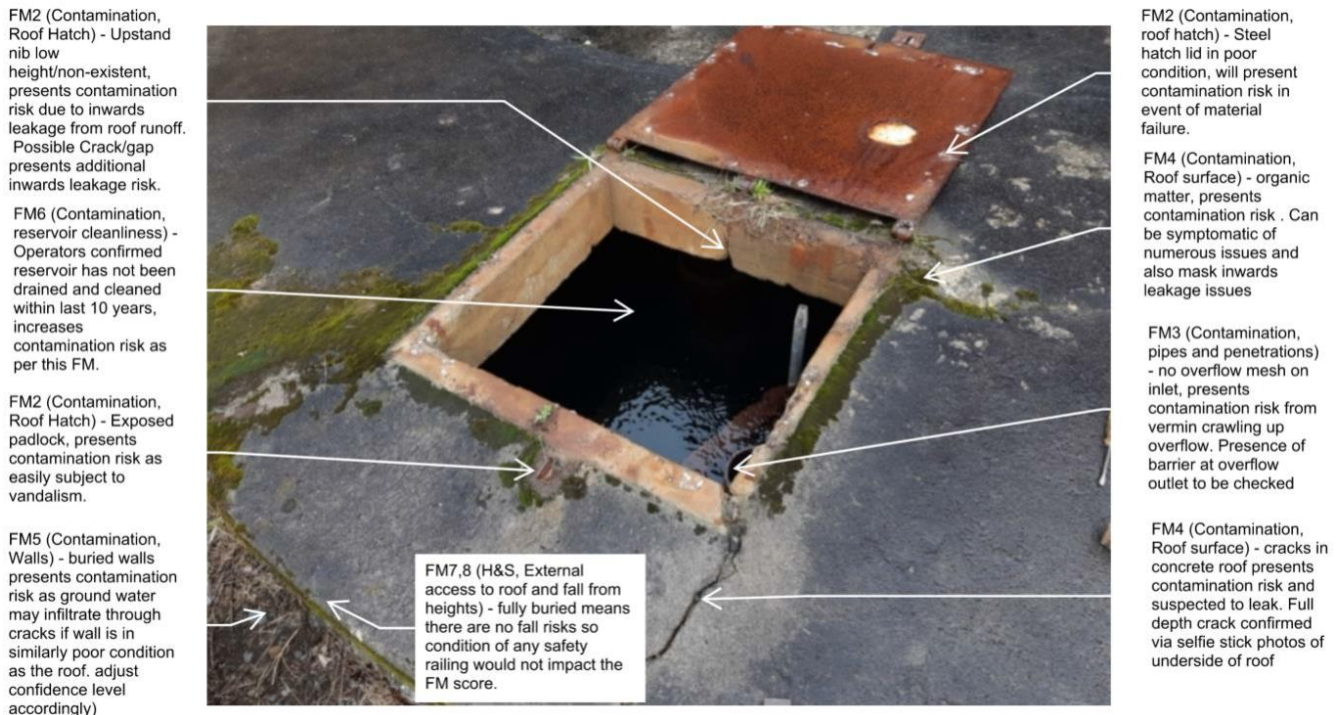
Figure 4 - Example of the typical 'thought process' that the field assessors needed to follow,
