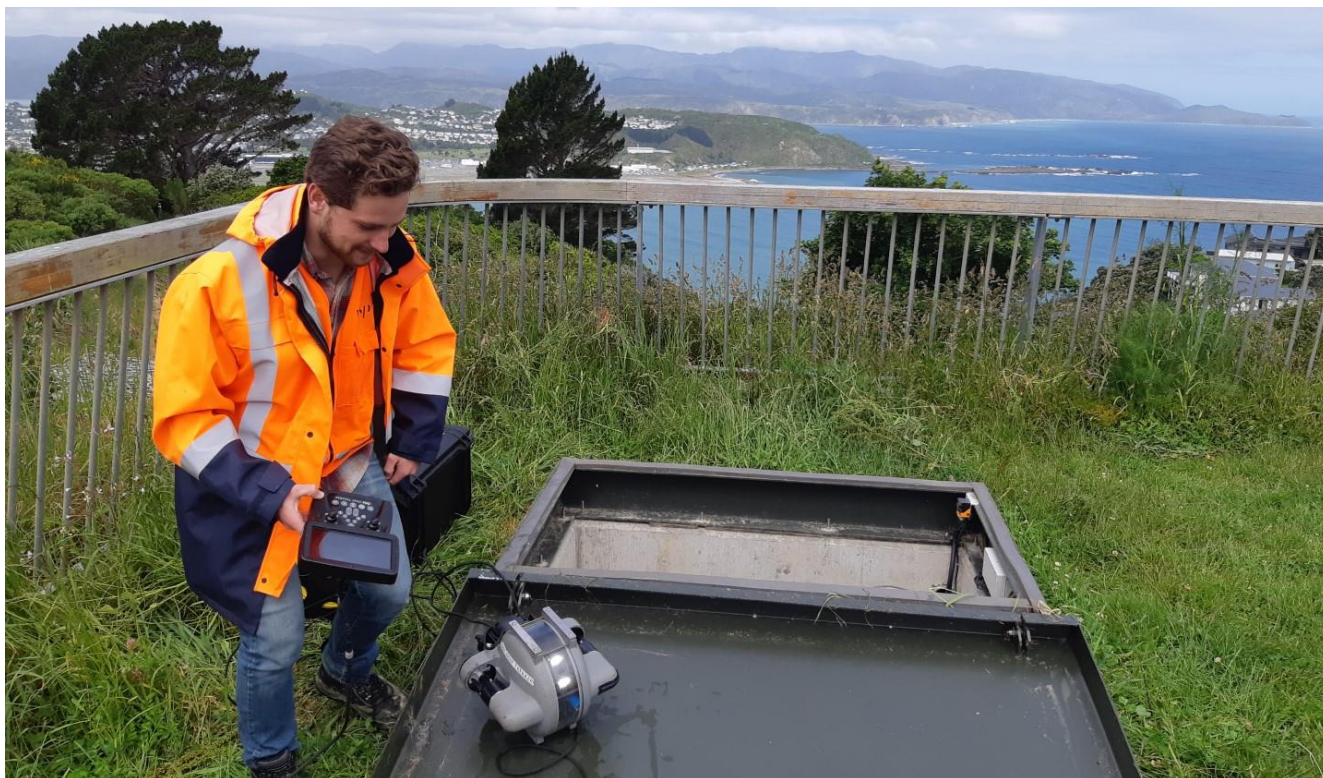
Figure 9 – Commencement of a submersible drone inspection.
