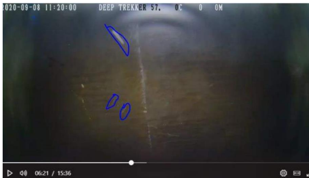
Figure 8 – Example of 'online' roof leakage testing
