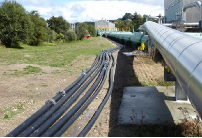
Photograph 3: Trial pipes; 100mm dia. x 200m, 150mm dia. x 400m
