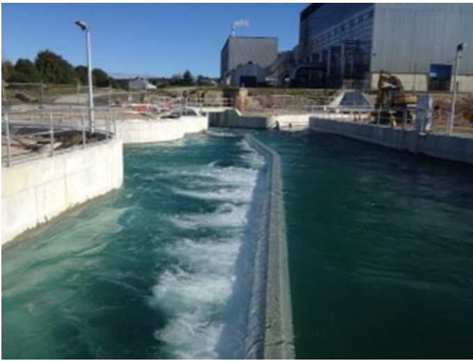
Photograph 6: Bypass side-weir on inlet channel
