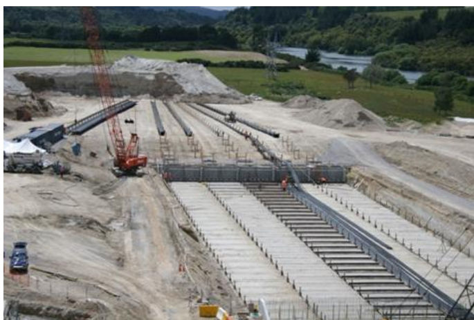
Photograph 7: Pulling 100m lengths of pipe into position. Photograph 8: Head chamber construction
