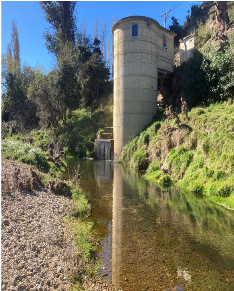
Figure 44: Waikouaiti Raw Water Intake Structure
