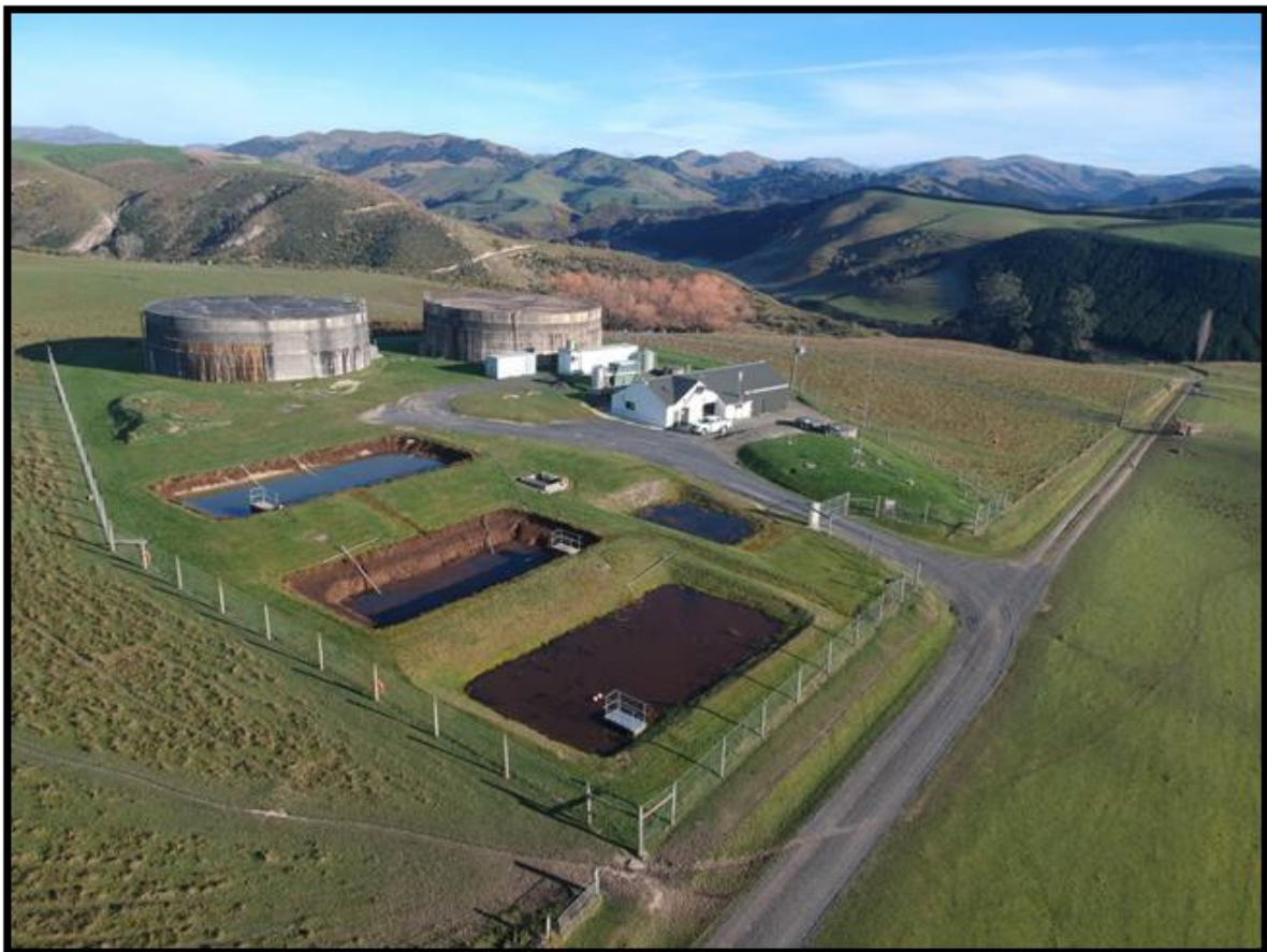
Figure 2: Waikouaiti Water Treatment Plant
