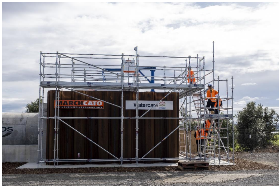
Photograph 3: Completed multi-purpose training facility
