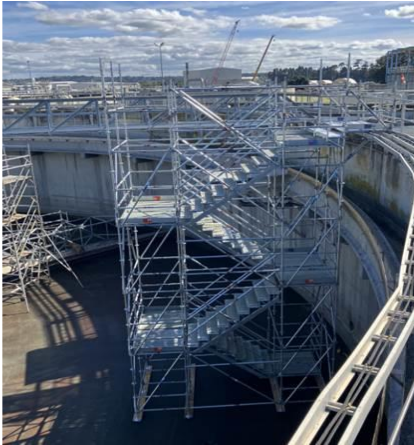
Picture 5. Scaffold tower with stairs installed in RC.
