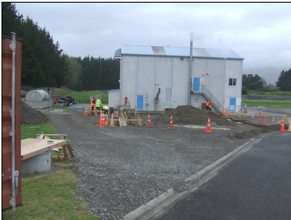
Photograph 3: Construction underway adjacent existing Sludge Drying Plant
