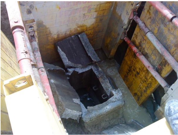
Photograph 1: Deconstruction of original brick arch manholes
