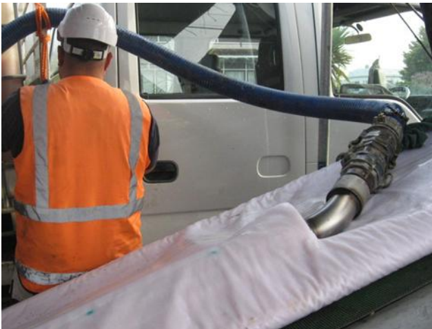
Photograph 5: Liner Impregnation with resin
