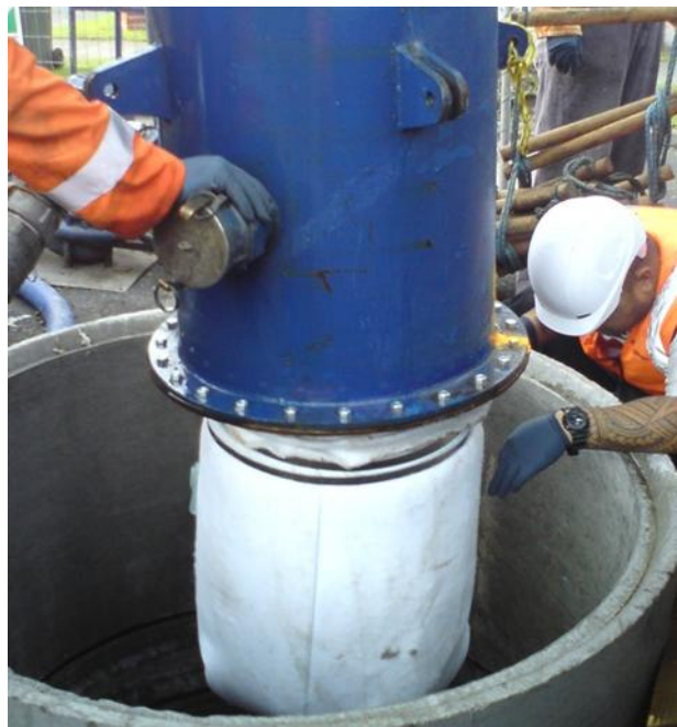
Photograph 8: Inverted liner ready for insertion
