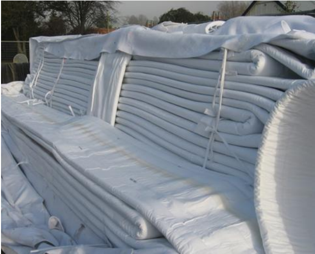
Photograph 3: Liner tubes delivered to site
