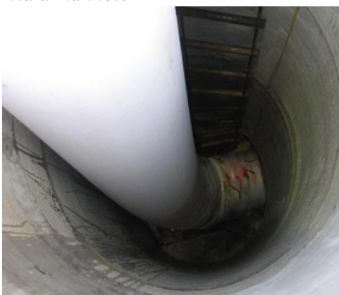
Photograph 9: Inverted liner full of curing water inserted into the pipeline via a manhole Photograph 10: Entire site set up within the centre of the road to ensure two-way traffic is maintained for the duration of the project.
