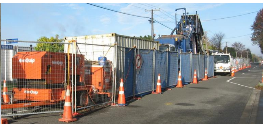
Photograph 9: Inverted liner full of curing water inserted into the pipeline via a manhole Photograph 10: Entire site set up within the centre of the road to ensure two-way traffic is maintained for the duration of the project.
