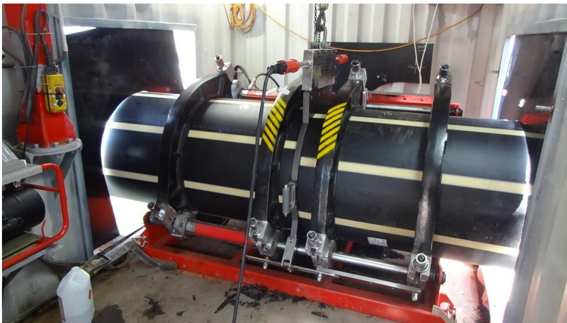
Photograph 6: Butt welding equipment at the site
