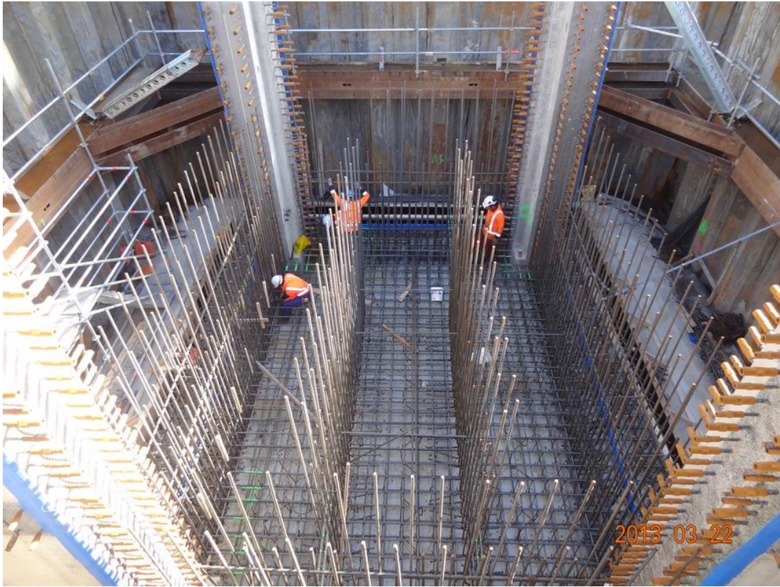
Photograph 3: Pump station wet well under construction
