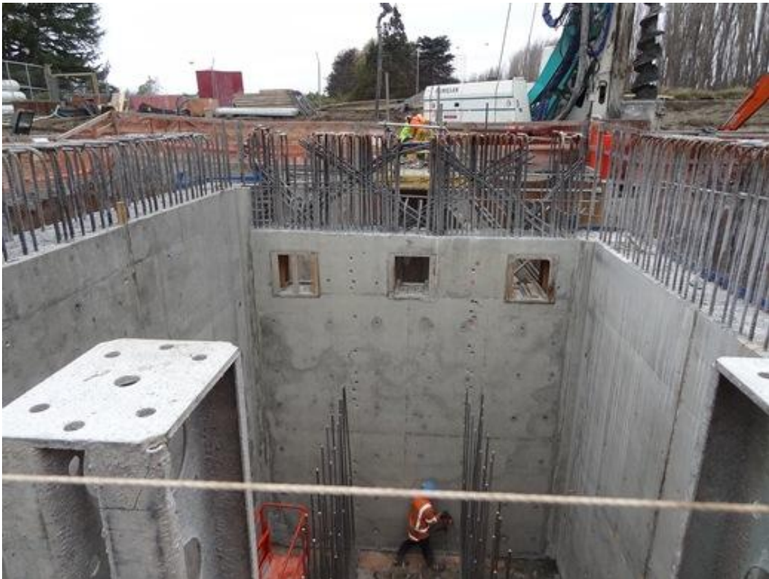
Photograph 3: Pump station wet well under construction
