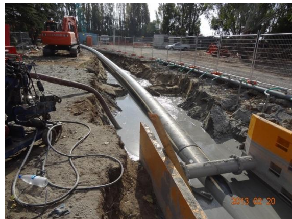
Photograph 5: Directional Drilling
