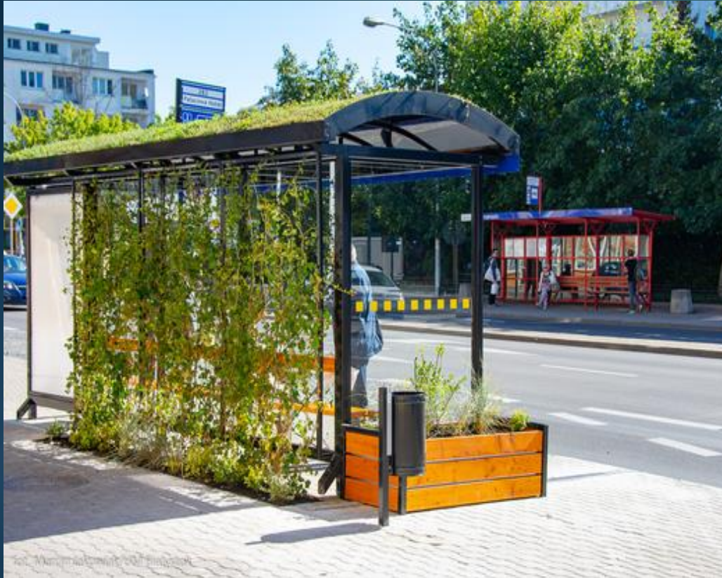
Living roof, green screen and planter box installation – Bialystok, Poland
