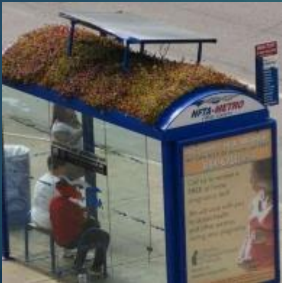
Living roof with solar panel – Buffalo, USA
