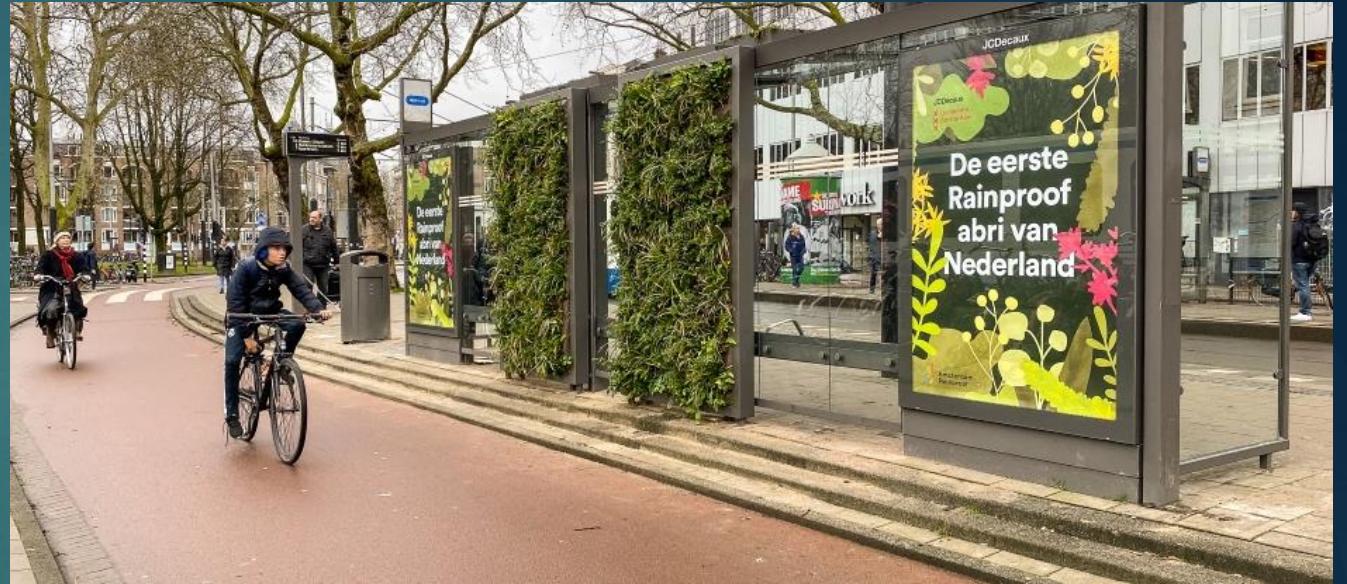
Living roof and greenwall installation – Wetering circuit at Vijzelgracht, Amsterdam
