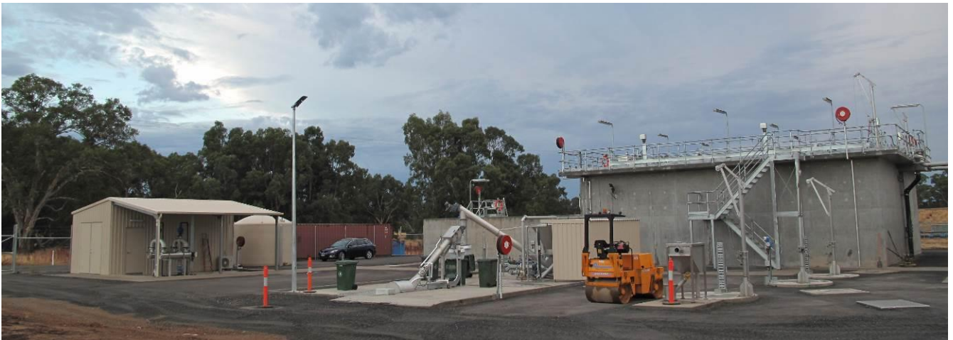
Photograph 3: UV system (left), inlet works (centre), SBR tanks (right)
