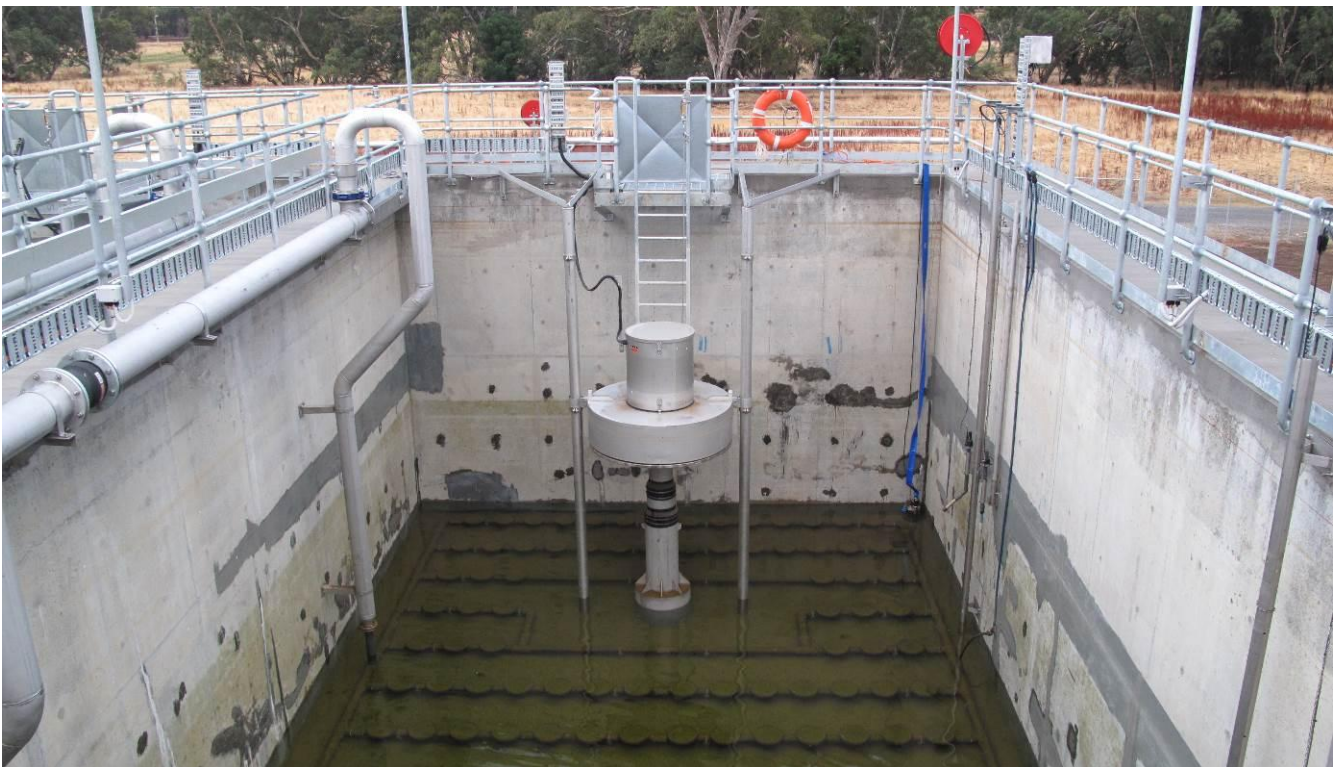
Photograph 4: SBR tank aeration grids prior to commissioning tests
