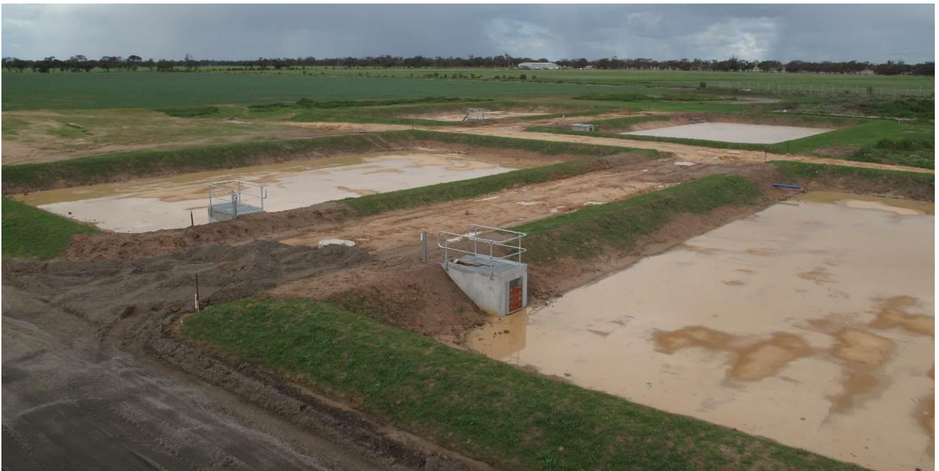
Photograph 11: Sludge drying lagoons
