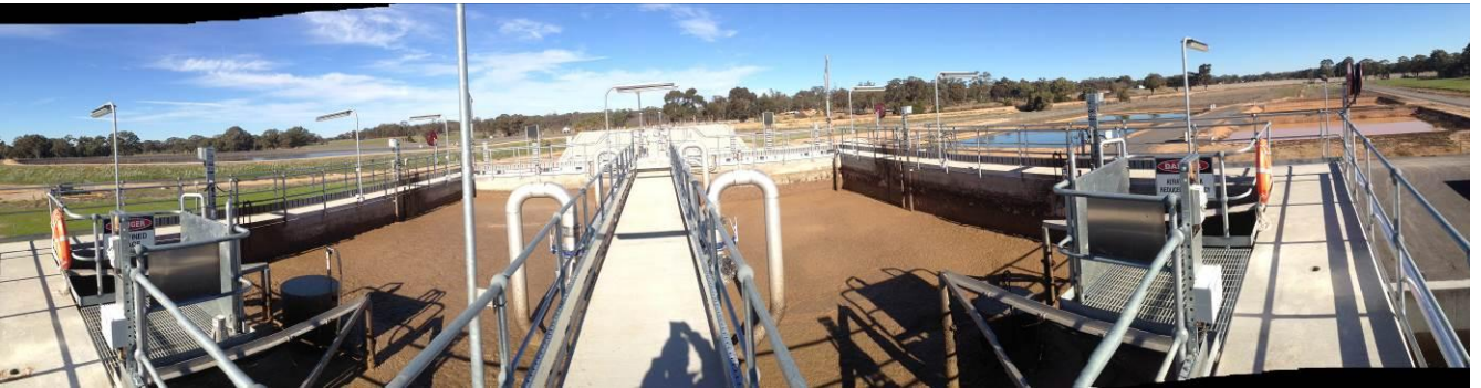
Photograph 8: SBR tanks (left and centre), and sludge drying lagoons (right rear)
