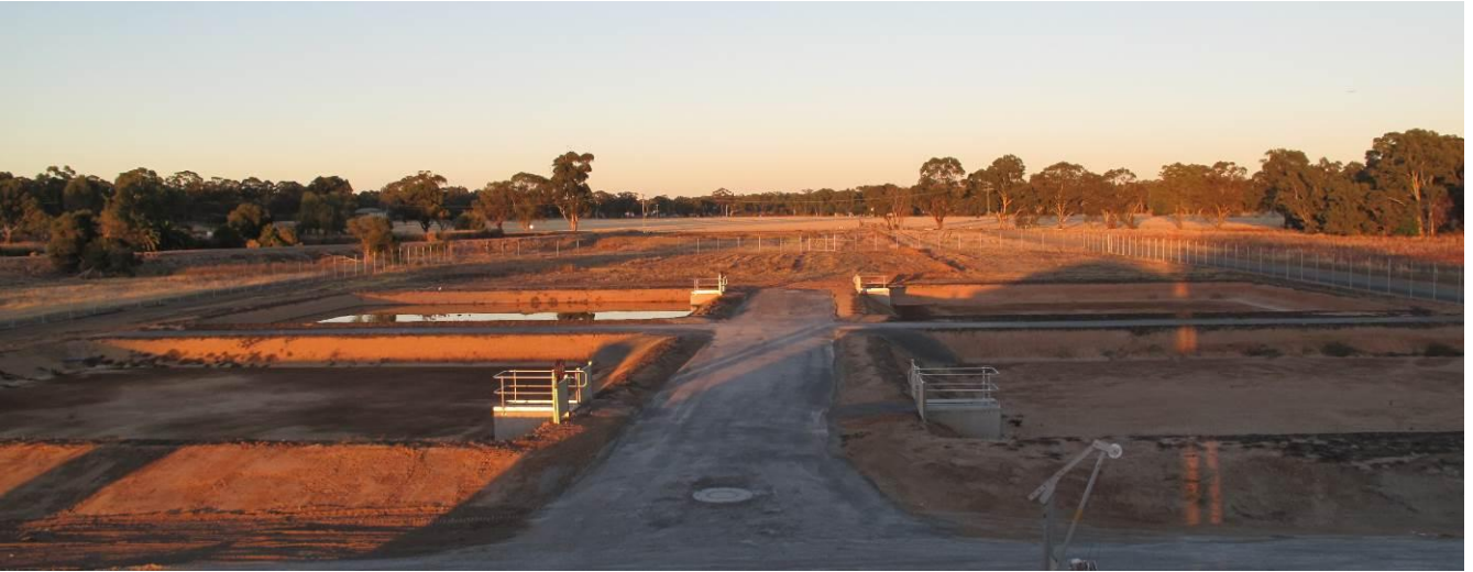
Photograph 5: Sludge drying lagoons
