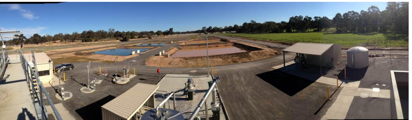
Photograph 9: Inlet works (foreground) and sludge drying lagoons (rear)
