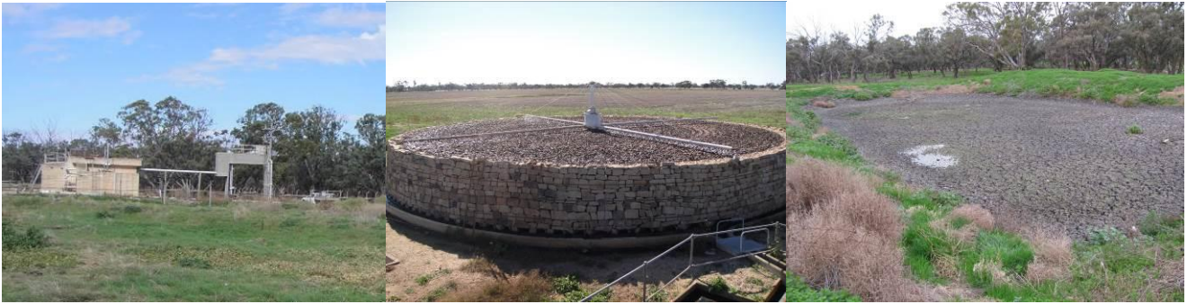
Photograph 2: Old Warracknabeal WRP From left to right; inlet and splitting structure, trickling filter, sludge lagoon
