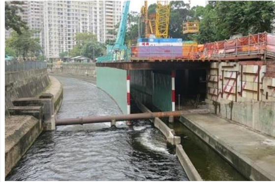
Erect temporary steel platform for piling works
