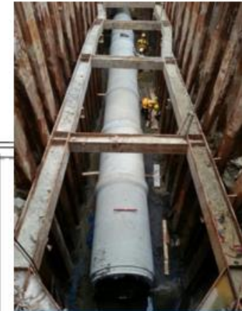
Construct 1200mm dia. sewer
