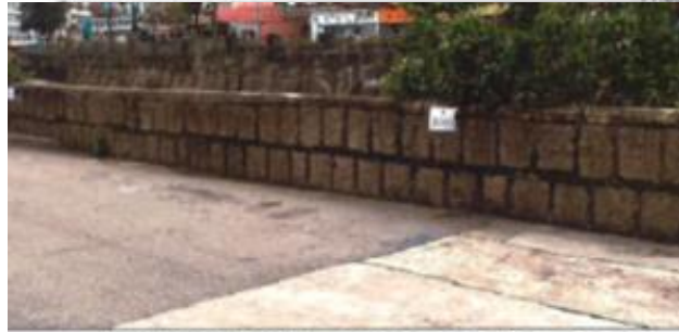
MASONRY WALL PHOTO (B360-B370)
