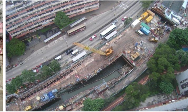
Erect temporary steel platform for piling works
