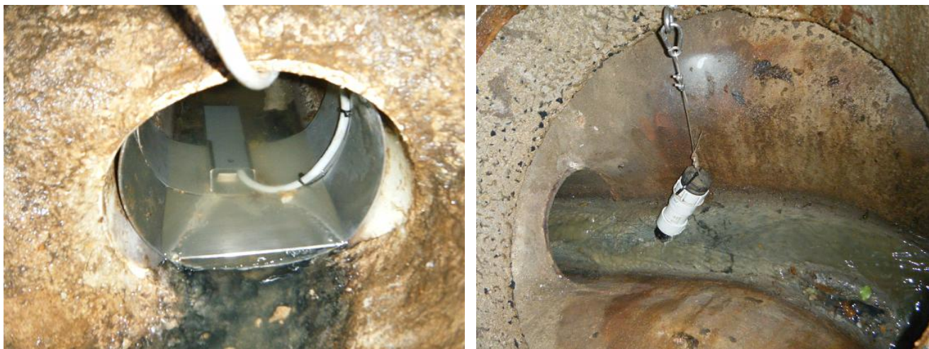
Photograph 2 and 3: Flow and conductivity monitor installations
