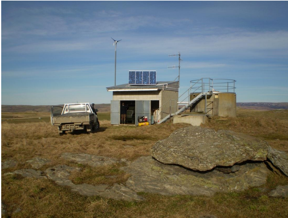
Photograph 1: Rocklands Water Treatment Plant
