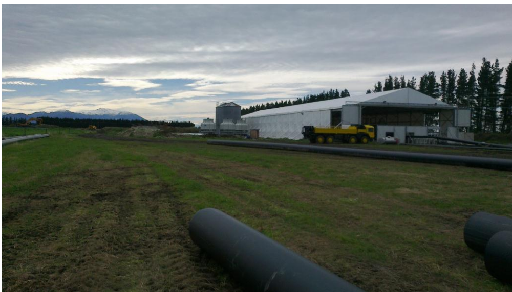
Photograph 4: On-site pipe manufacturing plant
