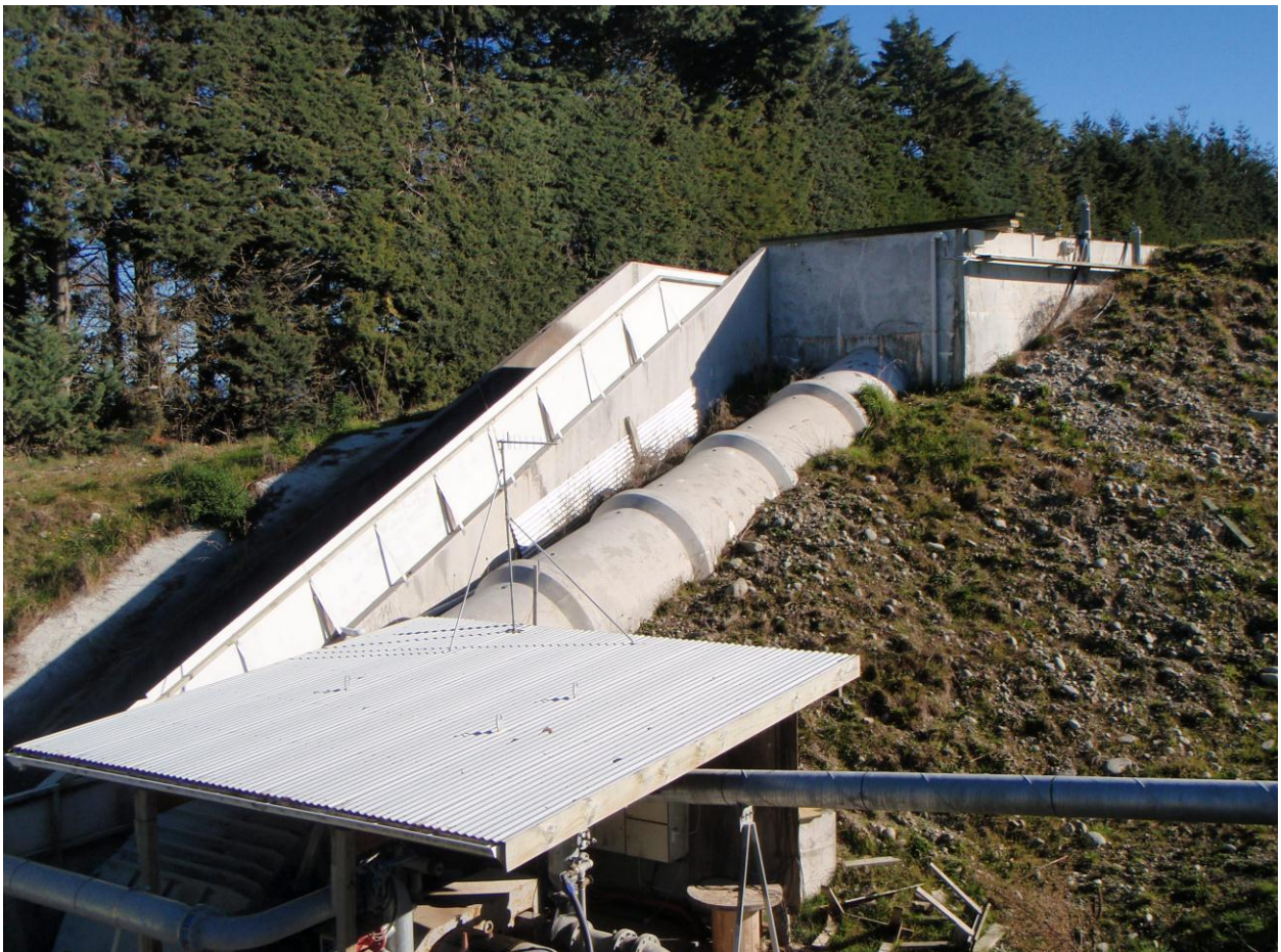
Photograph 5: An existing privately-owned hydro installation on the MHIS Main Race
