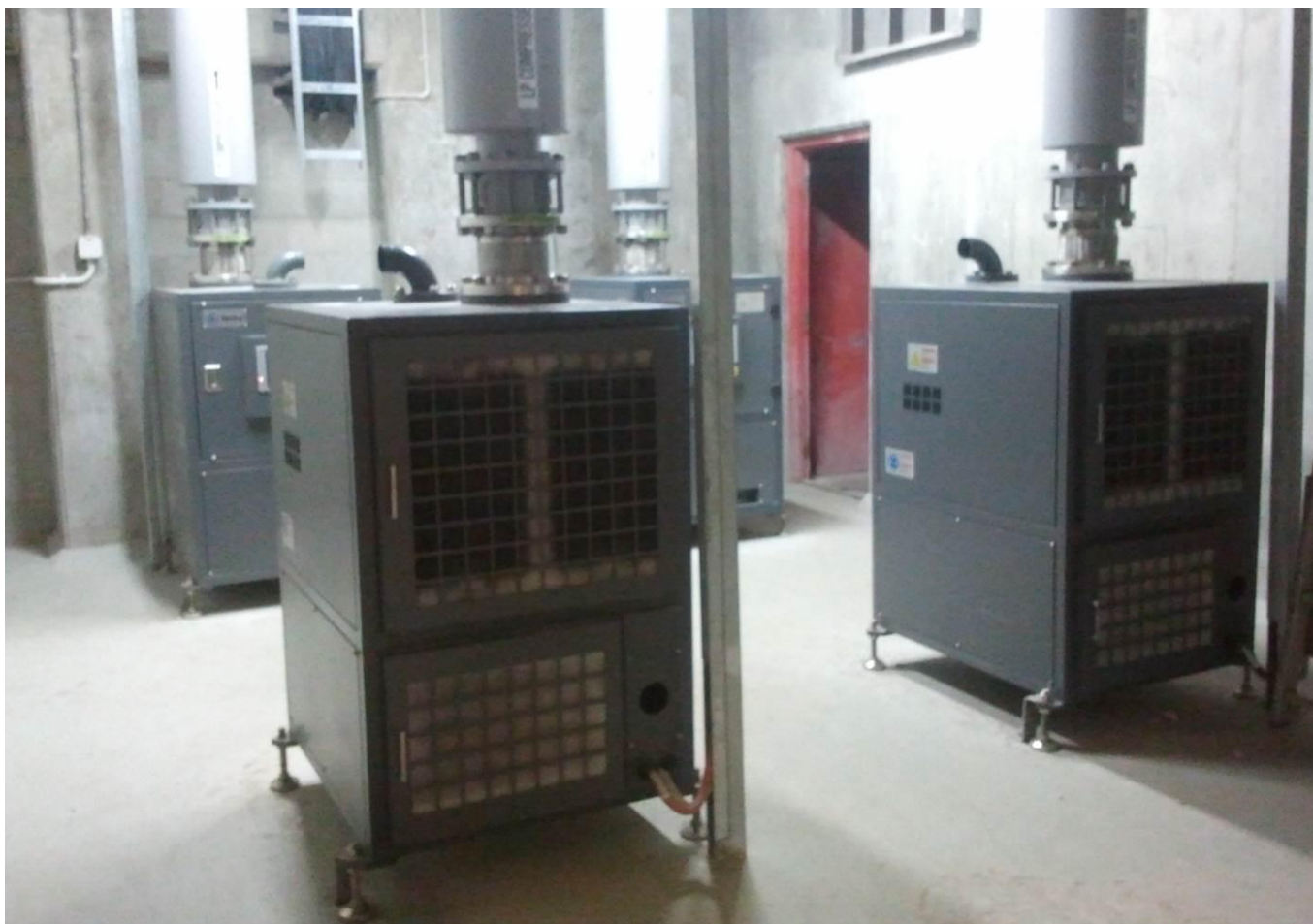
Photograph 2: K-Turbo High Speed blowers at Tahuna WWTP
