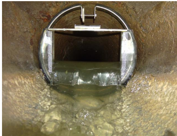
Figure 4: Portable Weir Installed in the Levin Trunk Sewer
