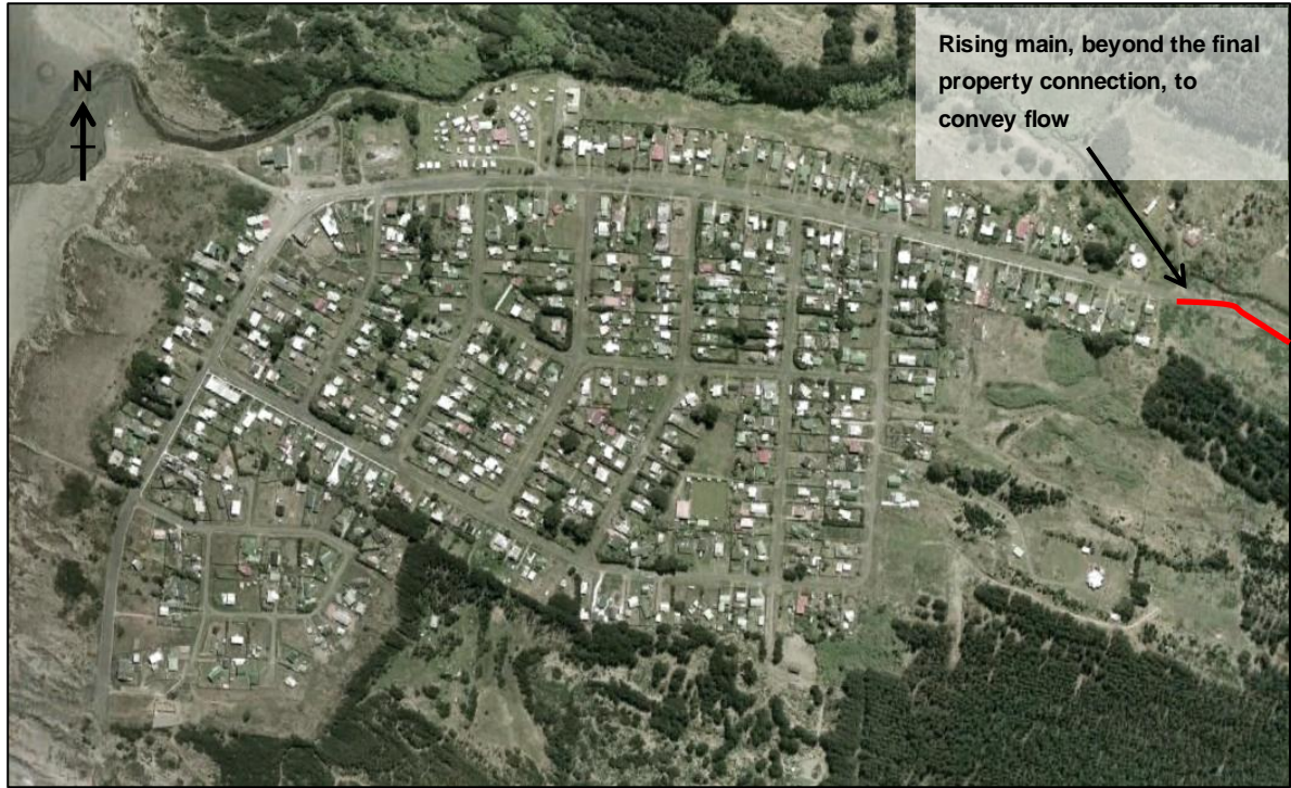
Figure 1: Aerial photo of Himatangi Beach township, showing the beach to the left (west) and the starting point of the proposed rising main shown to the right (east)
