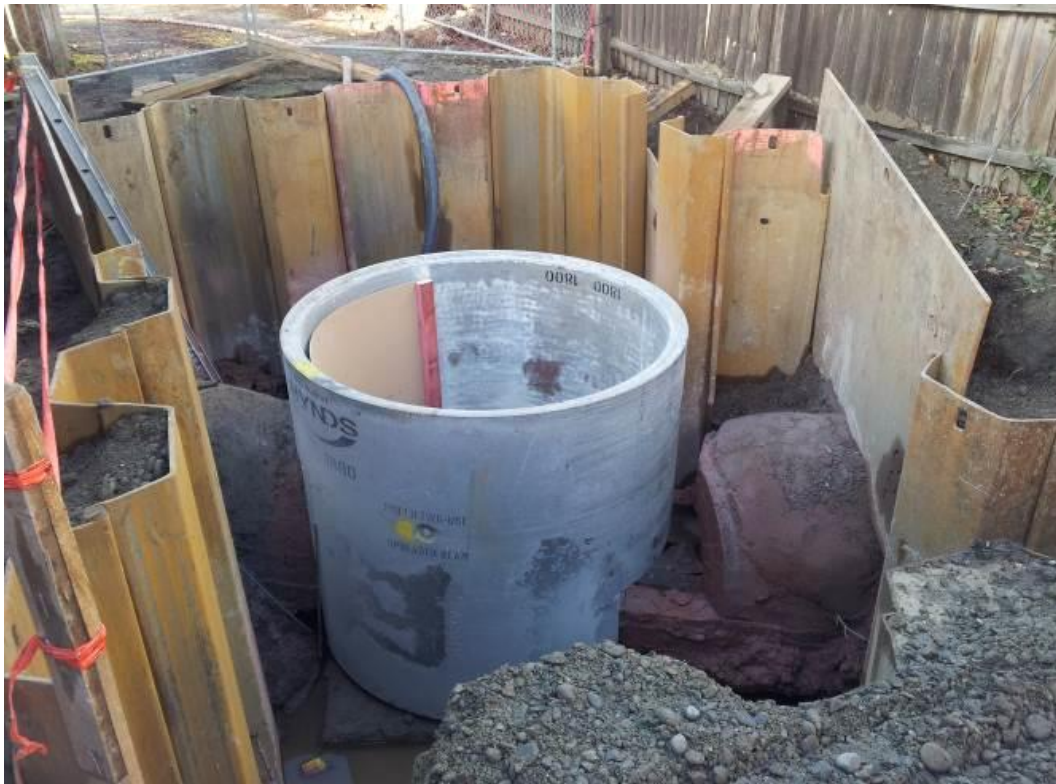
Photograph 12, New manhole construction with remaining brick barrel pipe exiting downstream
