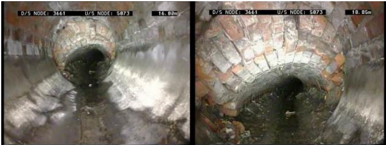
Photograph 4 and 5, Historic CCTV images of the collapsed pipe in January 2009 showed little difference
