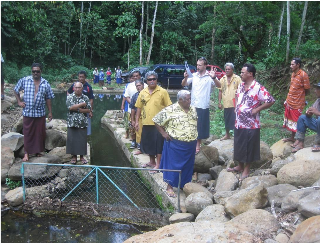
Photograph 7: Inspection of a community river intake.
