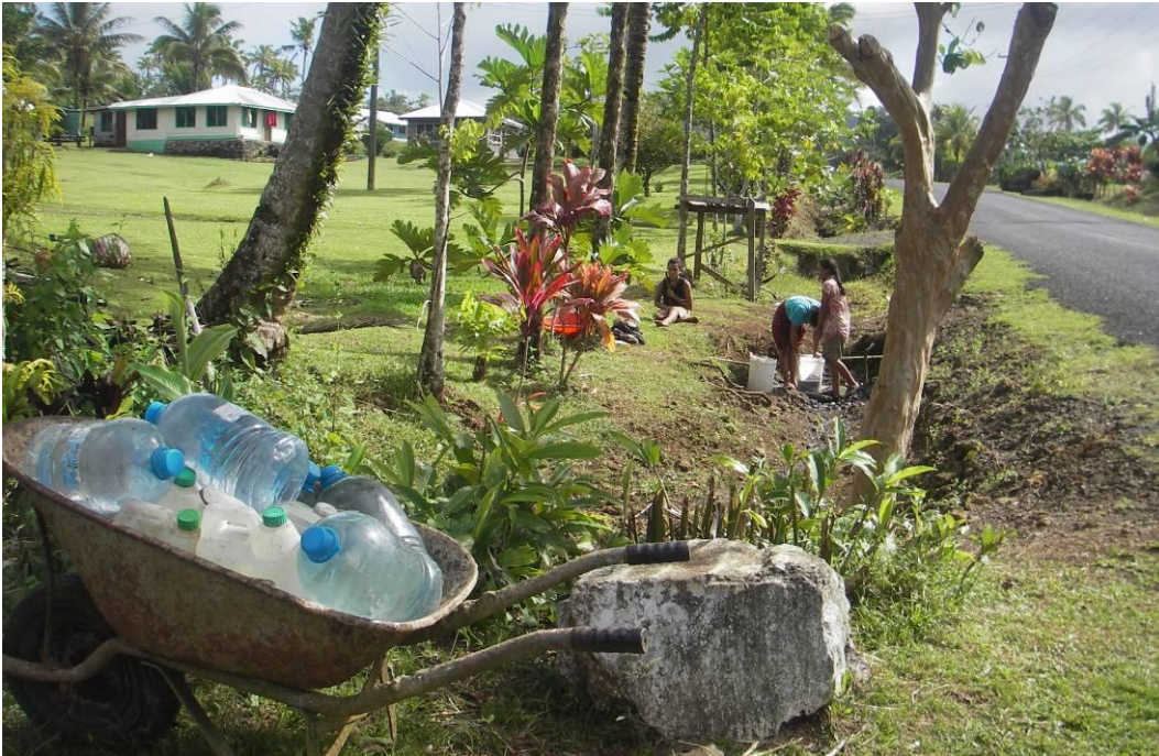
Photograph 2: Girls collecting household water from service pipe leakage.
