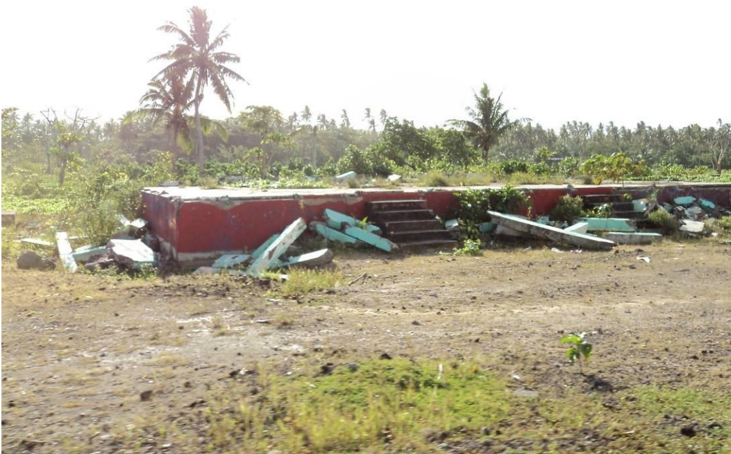
Photograph 4: Damage from the 2009 Tsunami – South East Upolu.
