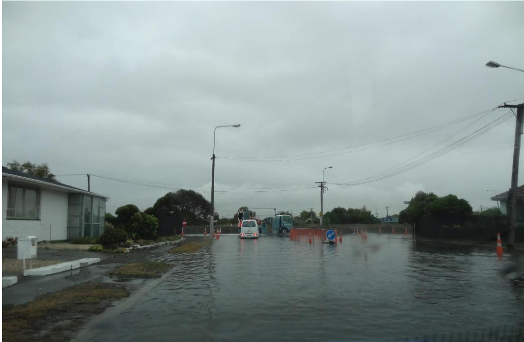
Photograph 1: Post-earthquake flooding on Beresford Street, New Brighton, in January 2013. Flooding was during a low intensity storm and high tide event, in a catchment that had experienced land settlement of up to 1.0m and severe damage to the stormwater reticulation
