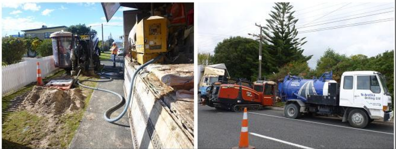
Figure 4 Installing street mains and property discharge line by trenchless technology
