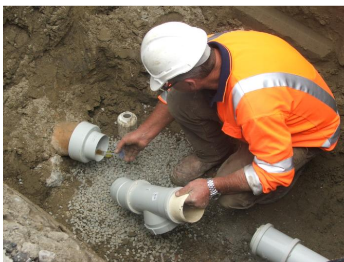
Photograph 8: Standard PVC fittings installed onto segmented PVC sewer pipe.
