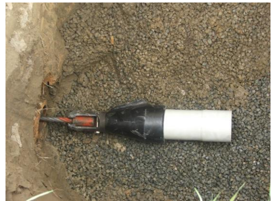
Photograph 3: Wire rope inserted connecting Pull-head with short starter pipe attached.
