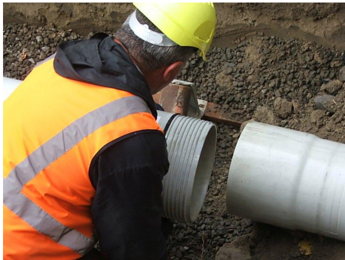
Photograph 1: Typical joint arrangement showing the rubber seal ring, threaded spigot and “low profile” threaded socket.
