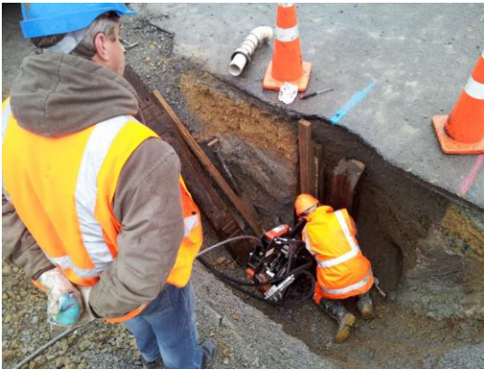
Photograph 2: Small compact Hammer Head PB30 to the ST-HY portable pipe burster in use.
