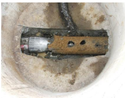
Photograph 6: Pull head passing through manhole...and, exiting manhole. Masterton
