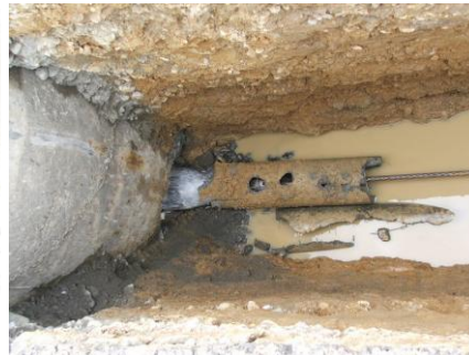
Photograph 6: Pull head passing through manhole...and, exiting manhole. Masterton
