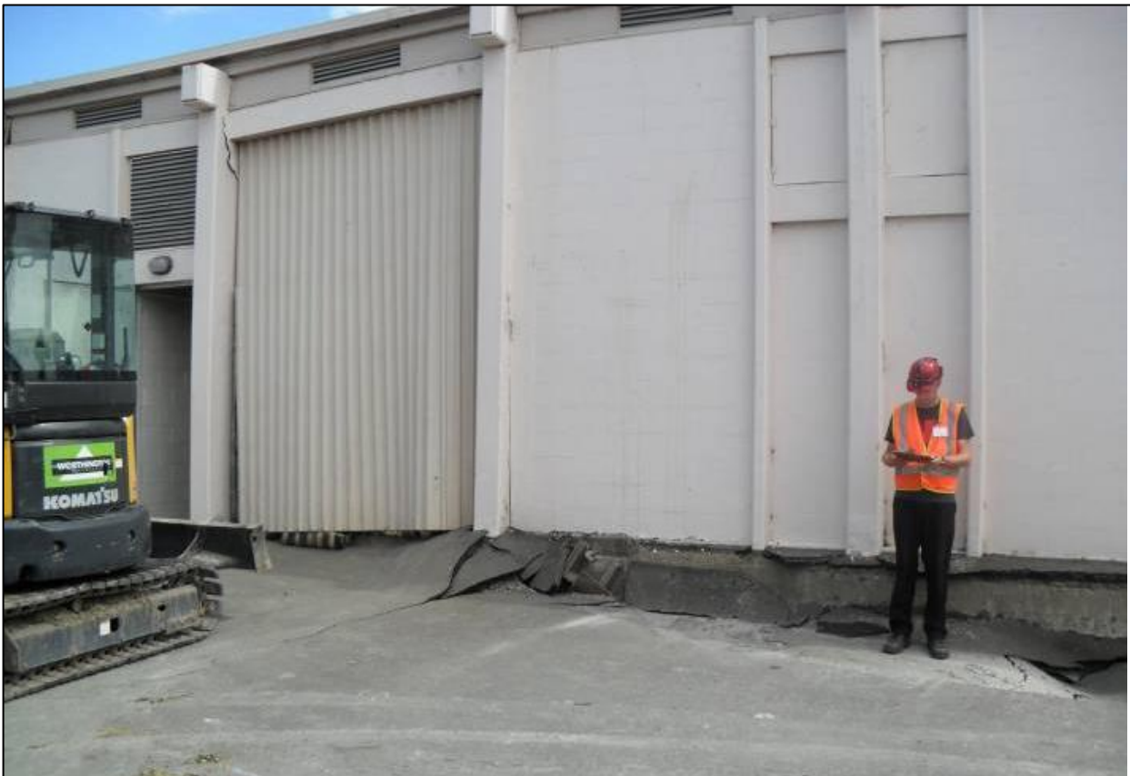
Photograph 1: Relative displacement of Caisson to ground level.
