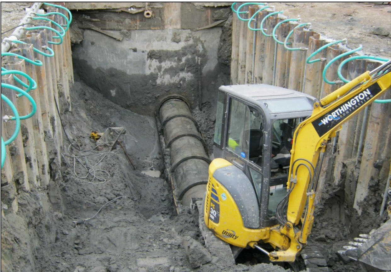
Photograph 3: Damage to caisson gravity pipe inlet (900 mm) showing pull out at connection to structure.
