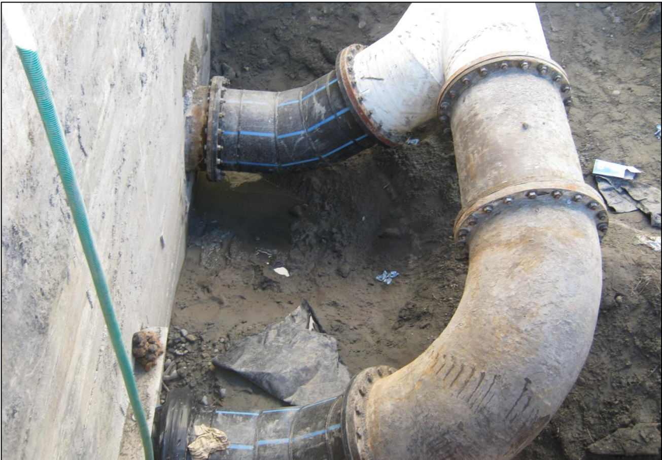
Photograph 9: Post-June 2011 Repairs to Pressure pipe outlet.
