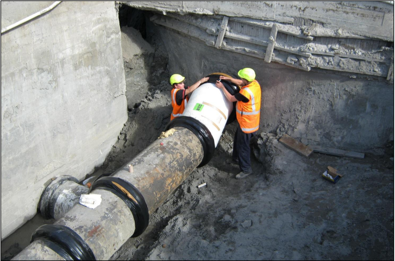
Photograph 9: Post-June 2011 Repairs to Pressure pipe outlet.
