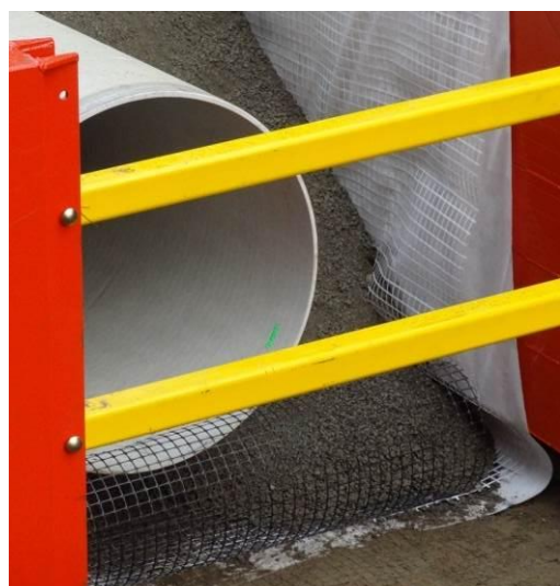
Photograph 3: Embedment installation
