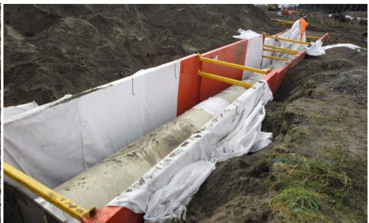
Photograph 5: Installation of pipes for testing
