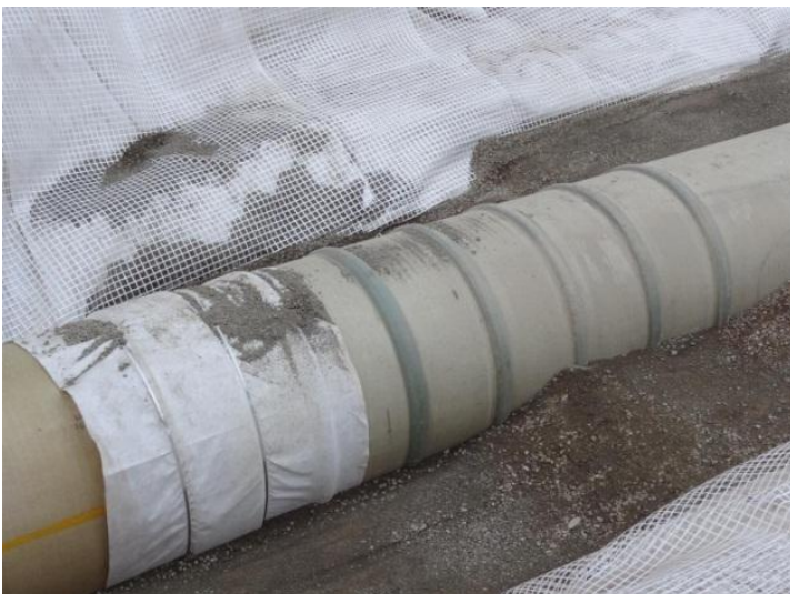
Photograph 2: Geotextile sock over coupler
