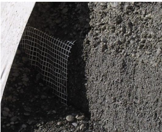
Photograph 4: Geogrid embedment wrapping
