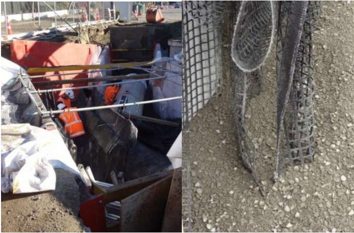
Photograph 1: Thrust block installation
