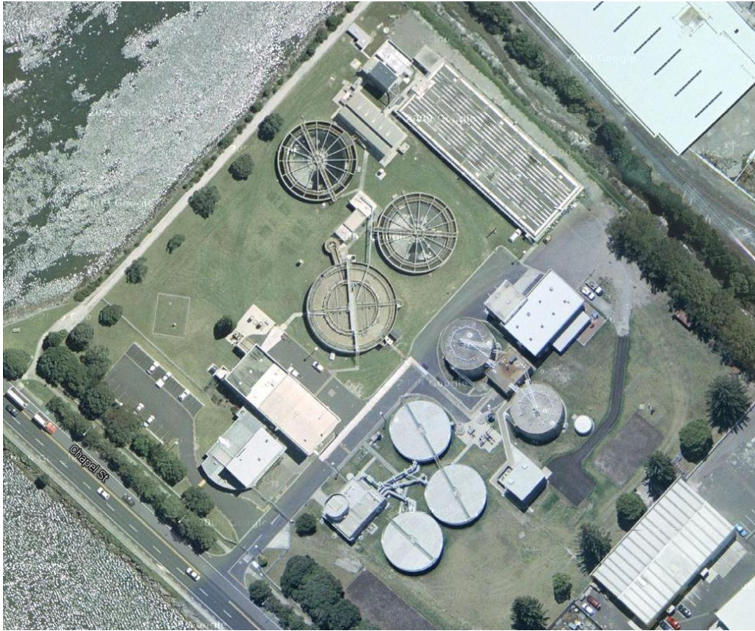
Photo 1: Aerial view of the Chapel Street WWTP 1
