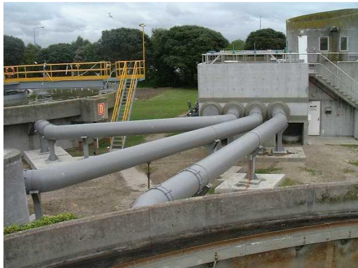
Photo 2: New pipework to feed the primary settling tanks
