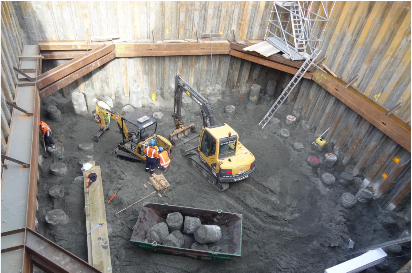
Photograph 2: CFA Piles at base of PS136
