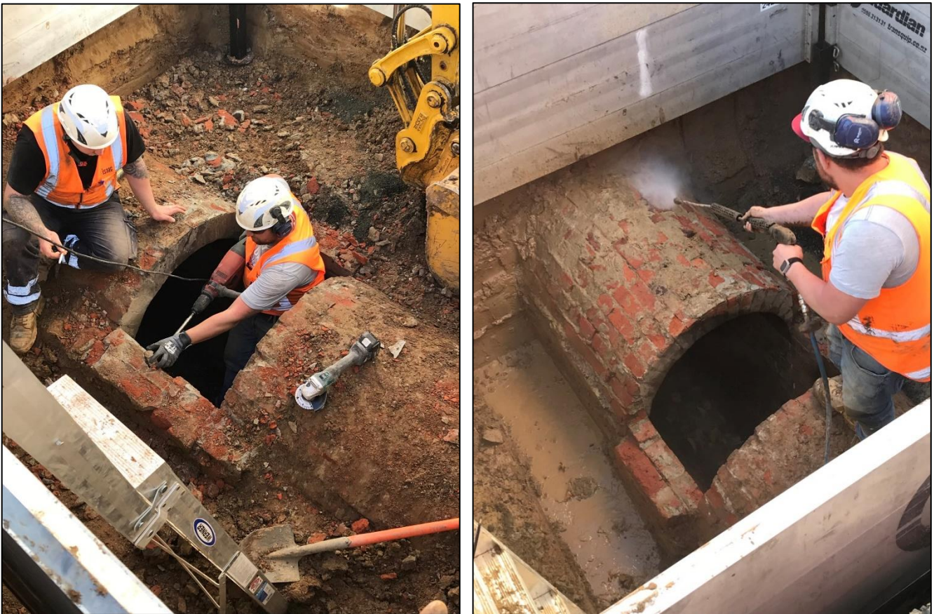
Photograph 2: Preparing the brick surface after removing the existing access
