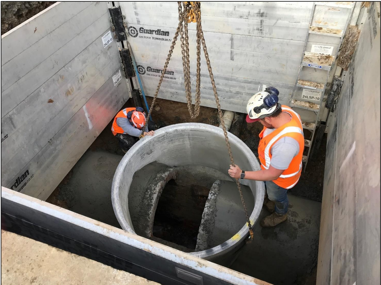
Photograph 4: Installing new manhole riser with semi-circular core on brick barrel
