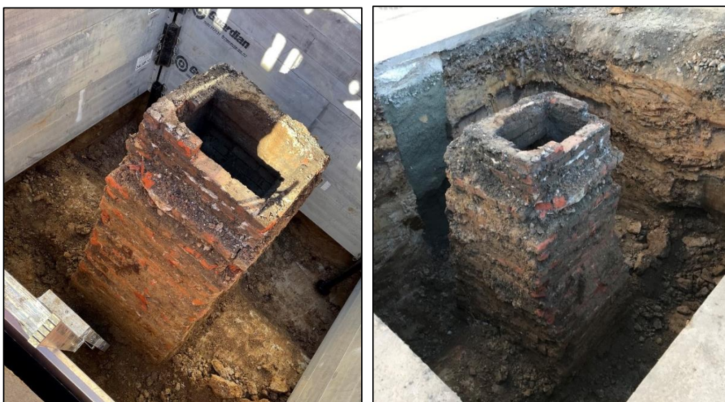
Photograph 1: Photos of exposed existing brick barrel access structures
