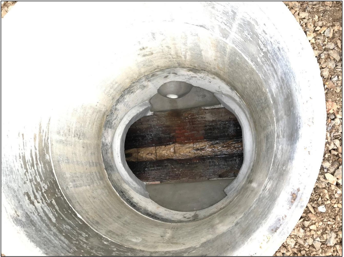
Photograph 5: Installing benching and additional manhole risers
