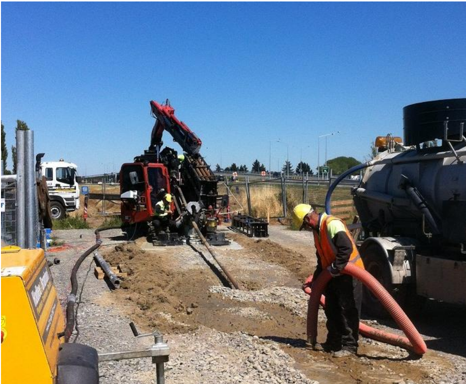
Photograph 1: Directional Drilling Operations
