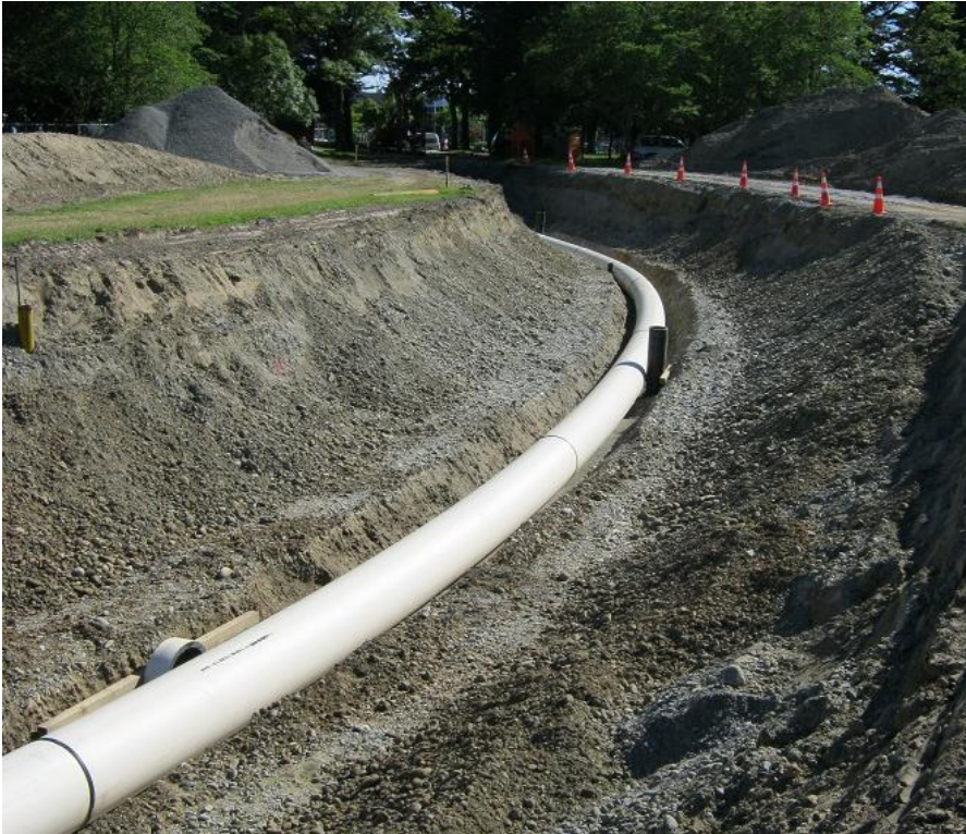
Photograph 2: Open Cut construction on a 'green-field' site
