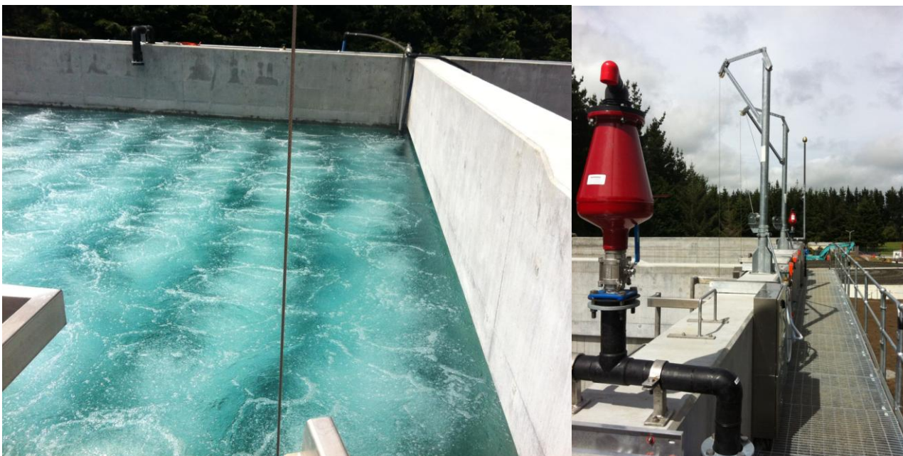
Photograph 2: Water testing of the SBR tanks
