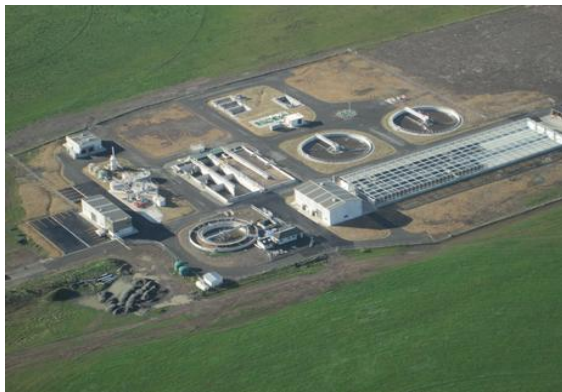
Photograph 3: Aerial View of Solar Drying Halls
