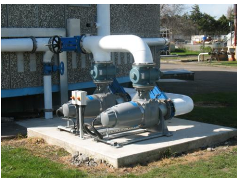
Photograph 1 and 2 Photo of External Mixing System (left) and Injector (right)
