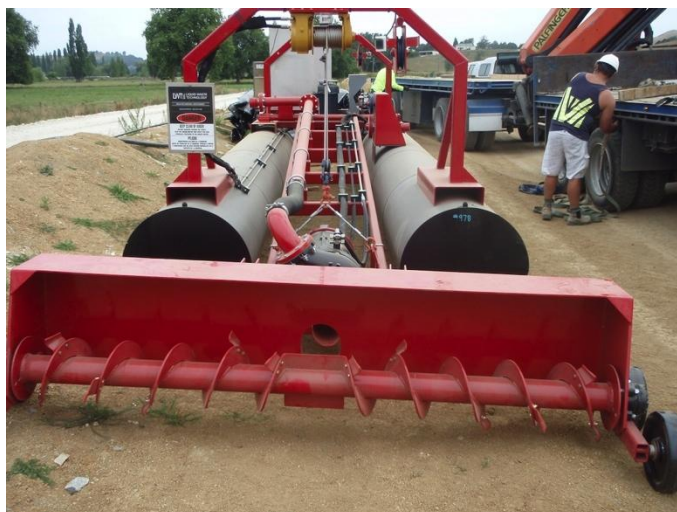
Photograph 14: Te Kuiti WWTP Dredge
