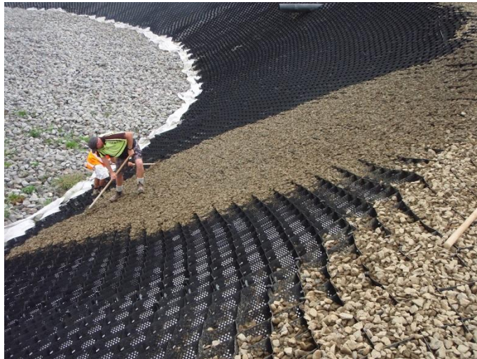
Photograph 3: Filling of Geoweb Erosion Protection
