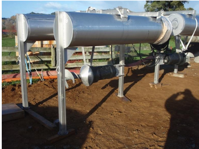
Photograph 6: Directional Floating Mixer
