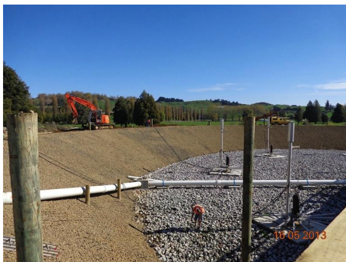
Photograph 4: Filled Geoweb Erosion Protection
