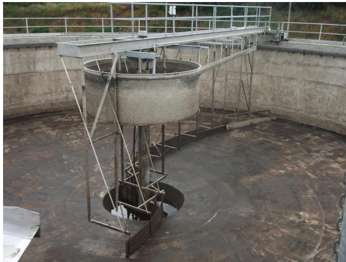
Photograph 13: Secondary Clarifier With Second Stilling Ring Installed
