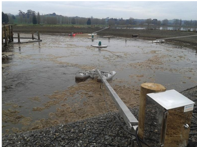
Photograph 7: Directional Floating Mixer in Operation
