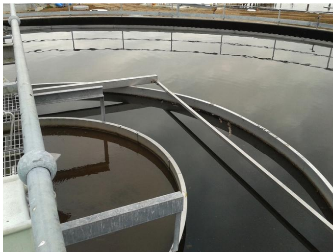
Photograph 13: Secondary Clarifier With Second Stilling Ring Installed
