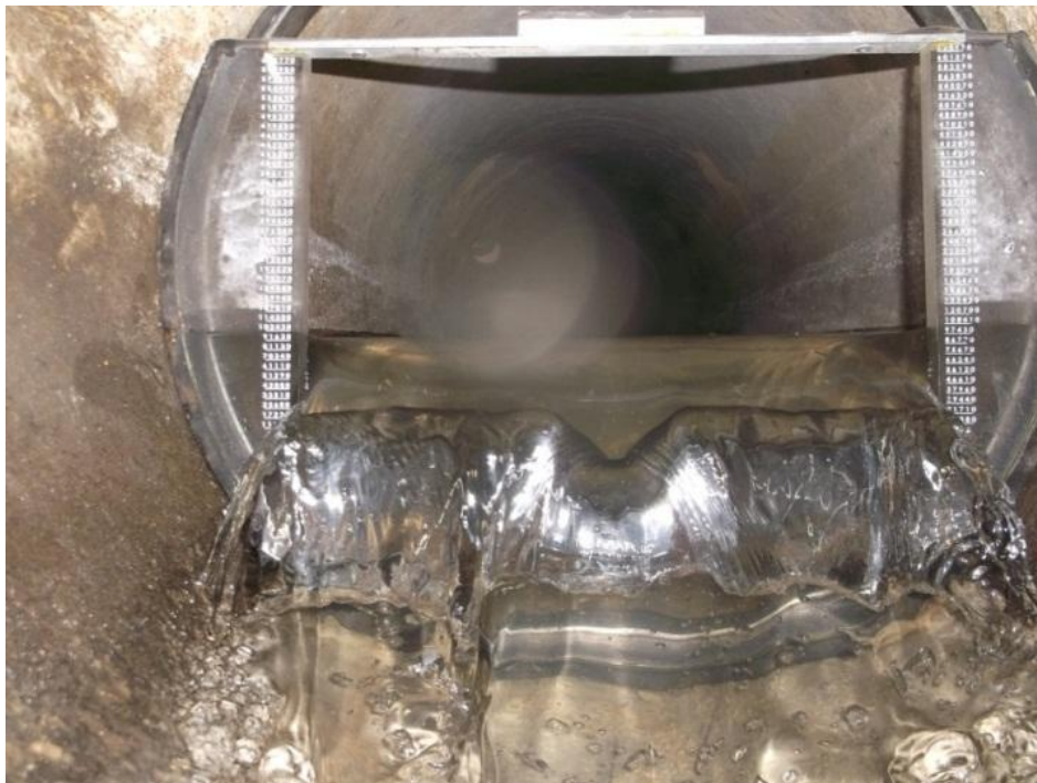
Figure 1: Portable weir installed in Featherston sewer
